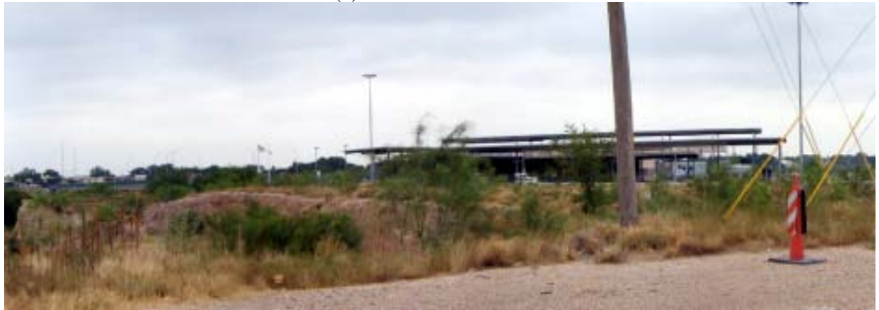
(b) View from the southeast
