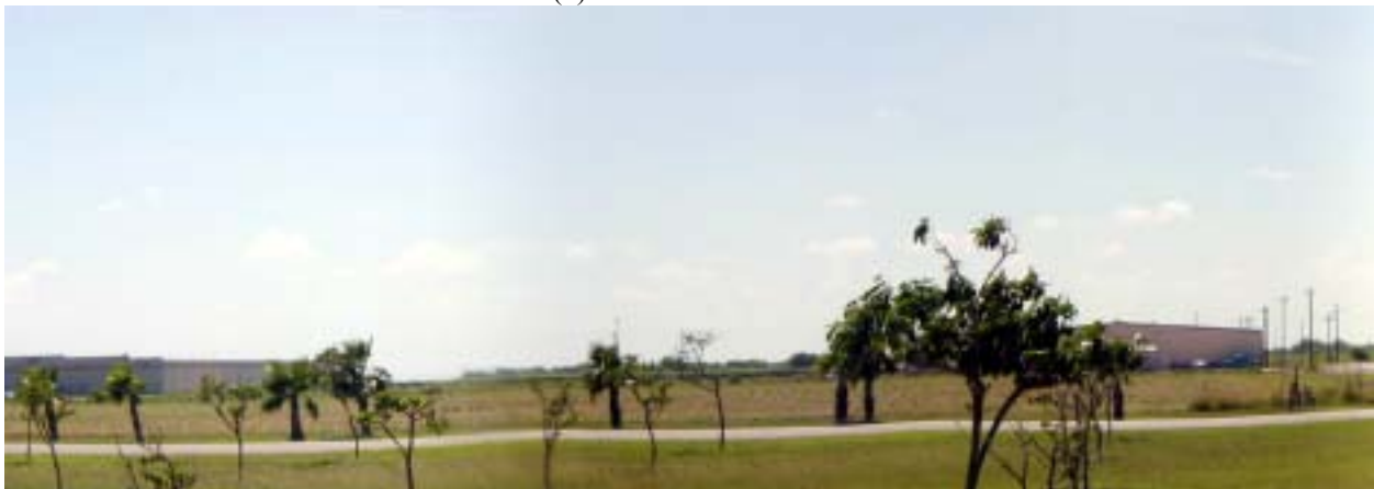
(b) View from the west
