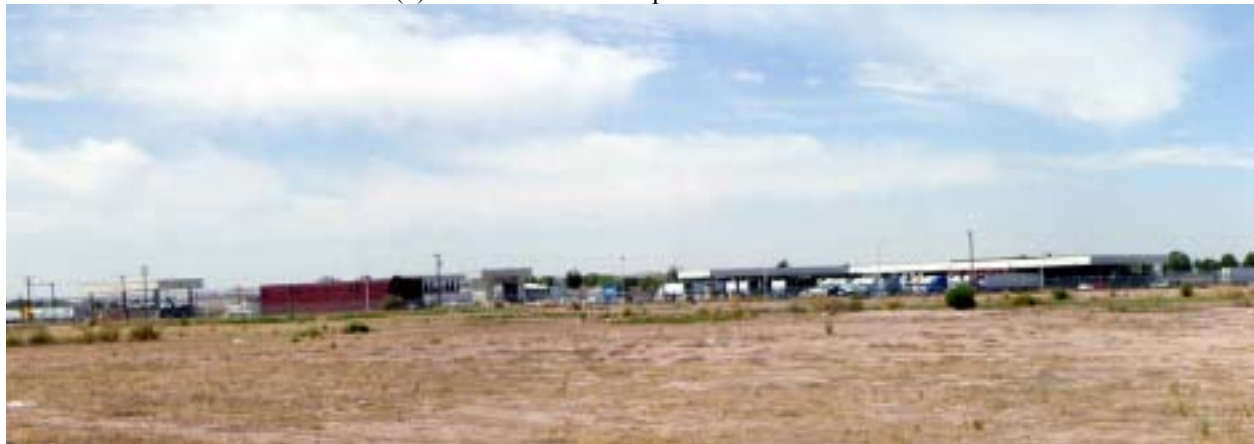
(b) View of federal compound from the east
