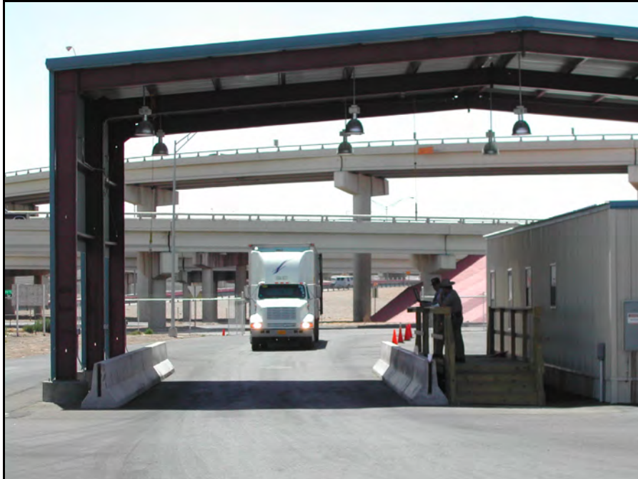
Figure 11: Truck Entering the DPS Commercial Vehicle Safety Inspection Facility at the Bridge of the Americas
