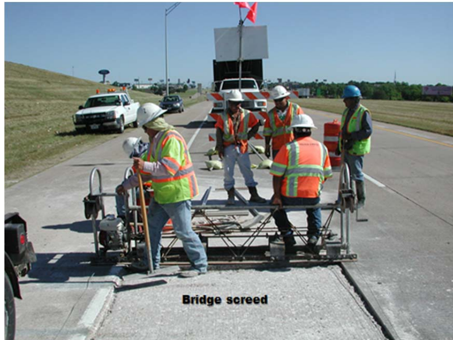
Figure 1.11: Bridge screed used to place thin application of concrete in southbound overlays did not work well on such thin overlays
