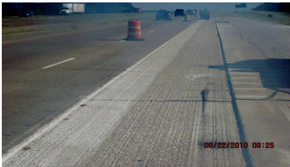
Figure 1.6: The depressed half of the faulted slabs was milled and overlaid
