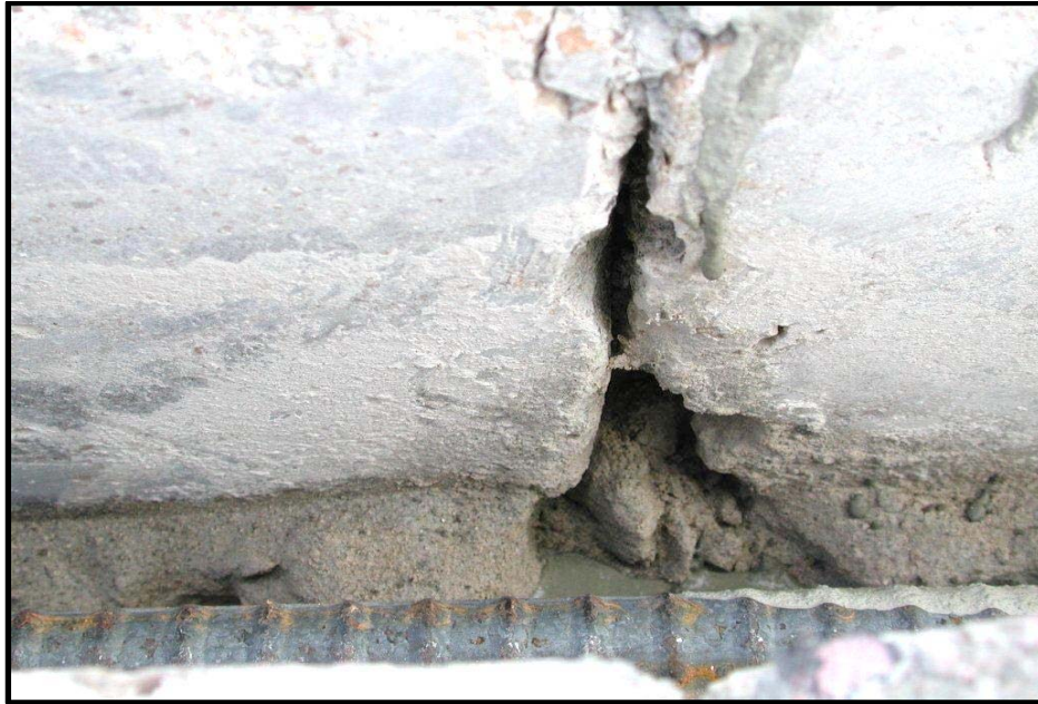
Figure 1.3: Unfilled voids mostly under unfaulted slab on the right.
