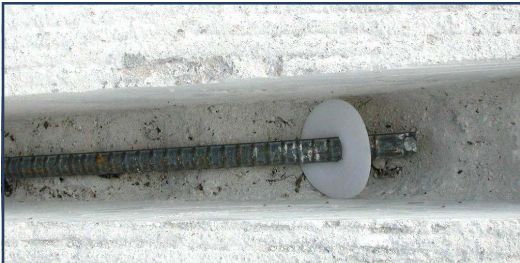
Figure 1.9: Plastic discs used for self-centering tie bar chairs
