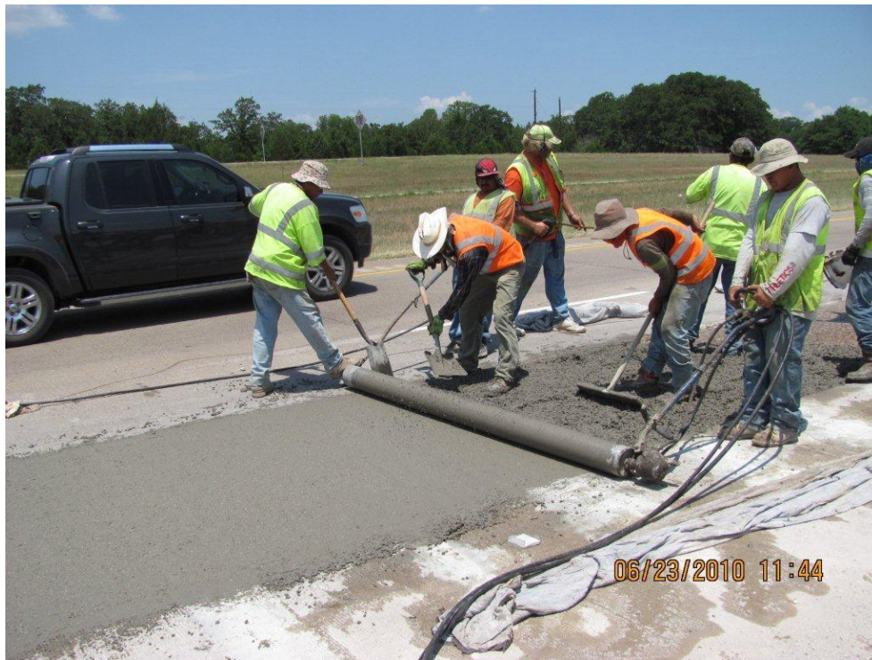
Figure 1.10: Rolling screed used on the northbound overlays worked well
