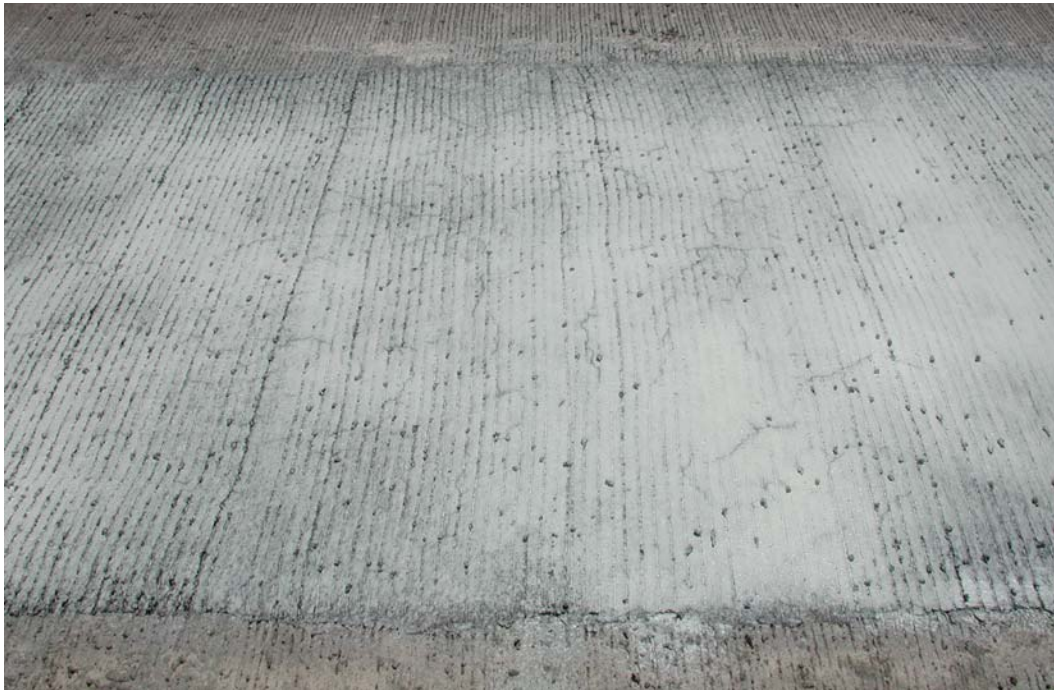
Figure 1.8: Early cracking in LMC overlay on southbound US 75
