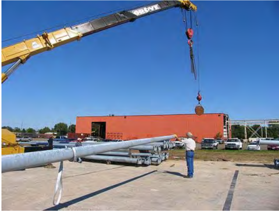
Figure 3 Crane Moving the 500-Pound Circular Weight to the Mast Arm End
