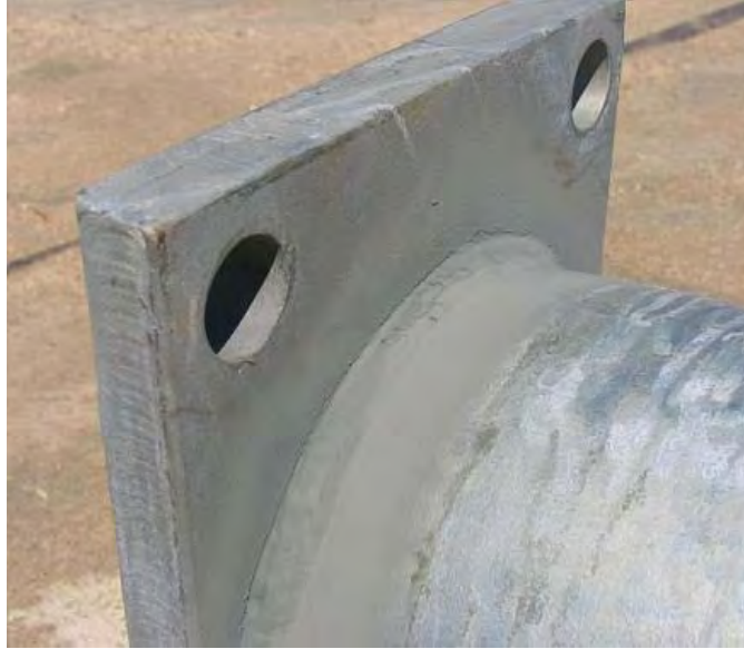
Figure 18 Mast Arm Weld After Completion
