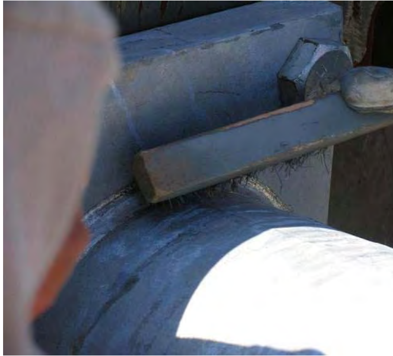
Figure 13 Removal of Galvanization with a Wire Brush
