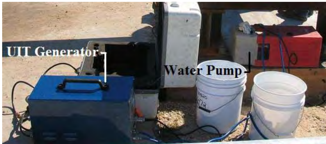
Figure 7 UIT Generator (Blue Box on Left) and Water Pump (Red Box on Right)
