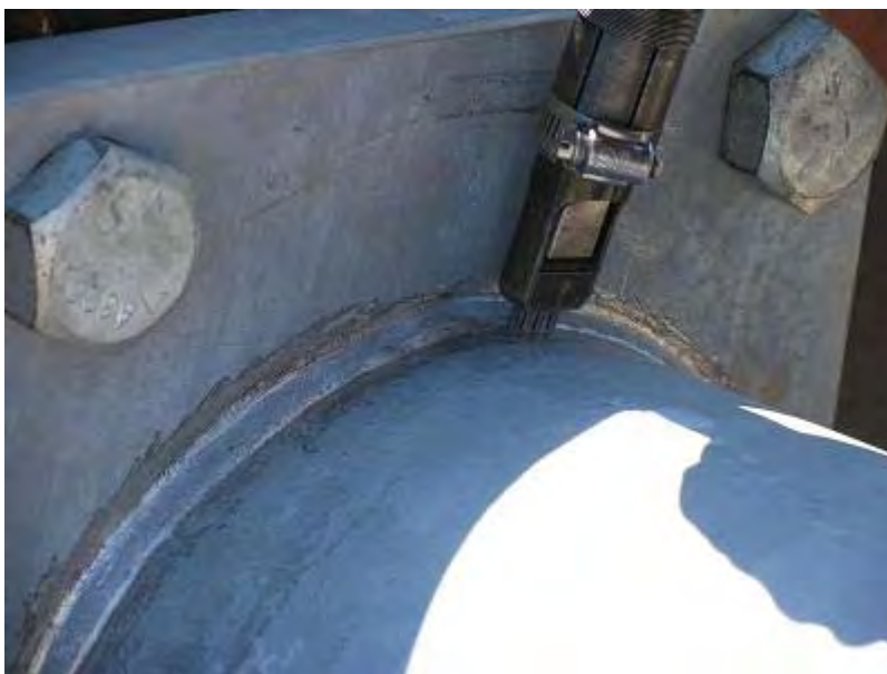
Figure 20 Employee's First UIT Application to a Mast Arm Weld
