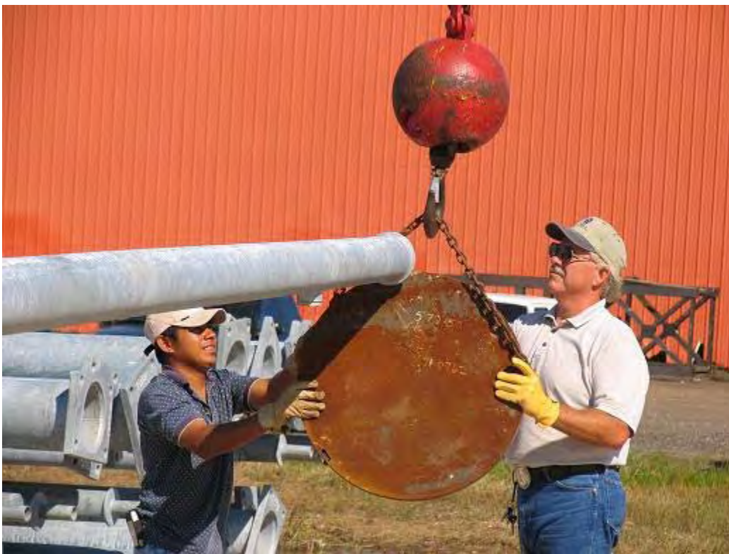
Figure 4 Placing the 500-Pound Circular Weight on the End of the Mast Arm
