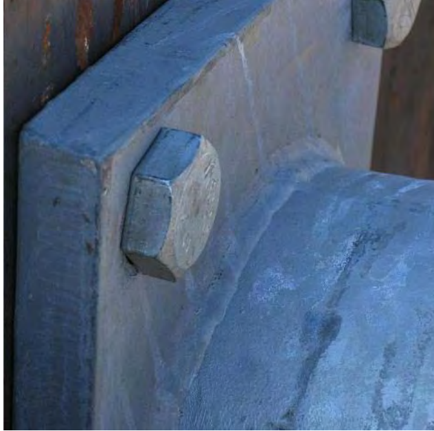
Figure 10 Mast Arm-Baseplate Weld Connection Before UIT Application
