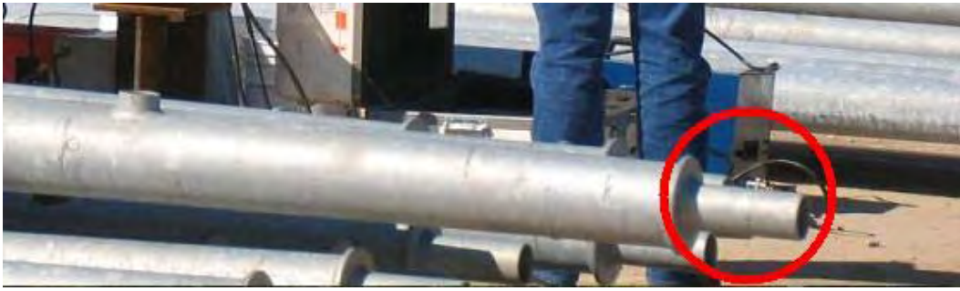
Figure 5 Mast Arm with 6-Inch Tenon at the End
