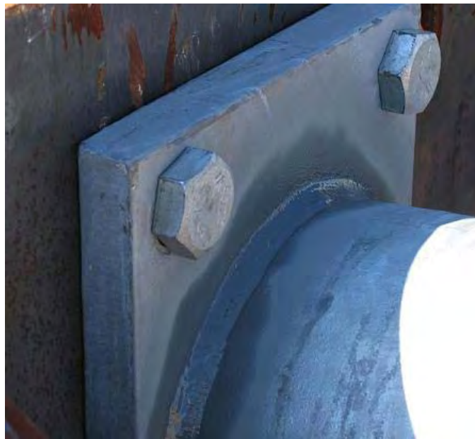
Figure 17 Drying Zinc-Rich Paint
