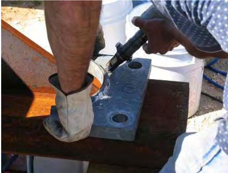
Figure 19 Employee Applying UIT to a Test Plate Weld
