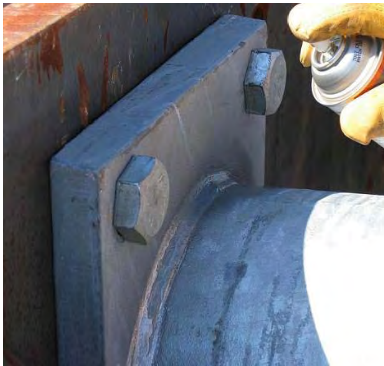
Figure 16 Application of Zinc-Rich Paint
