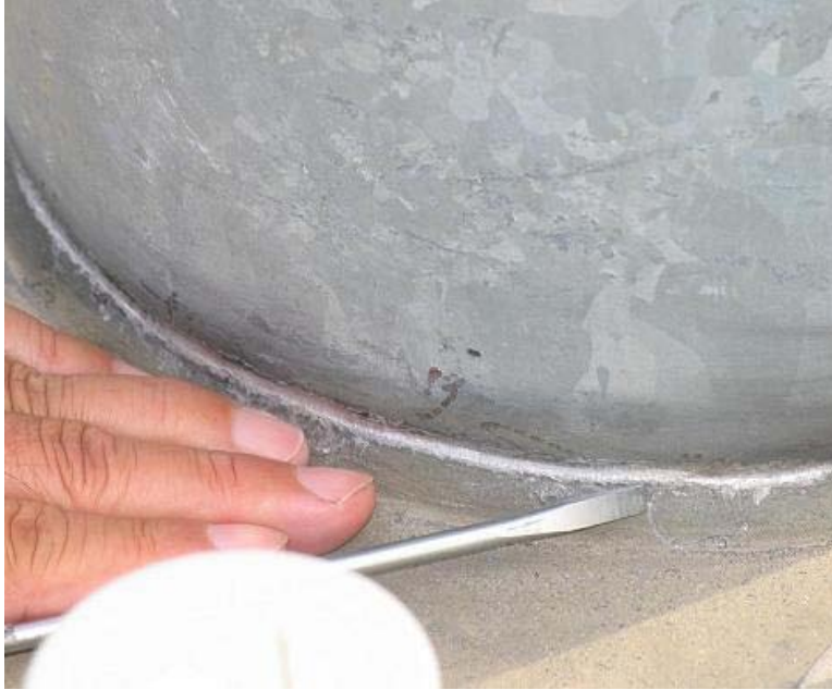
Figure 2.8 UIT Application at the bottom of Mast 2
