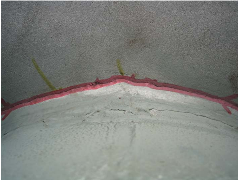
Figure 2.5 Fatigue Crack at End Plate Weld Toe in Laboratory Specimen
