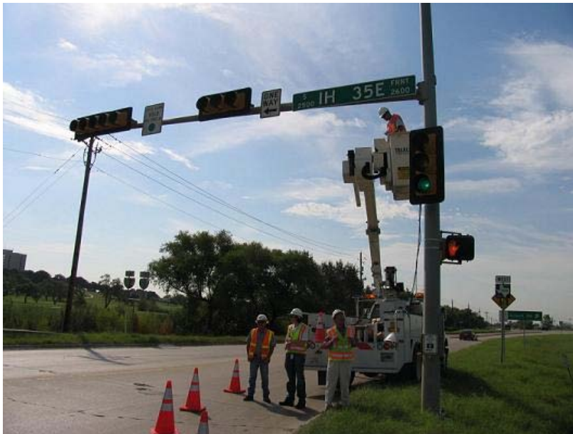
Figure 2.3 Mast Arm 2 at the Southwest Corner of the South Intersection of I-35E and Bonnie Brae Street in Denton, TX
