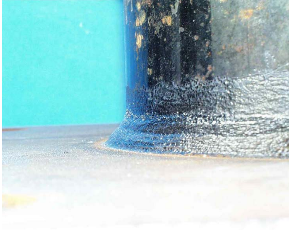
Figure 1: UIT Application to Both Weld Toes and the HAZ on TXuCLGP
