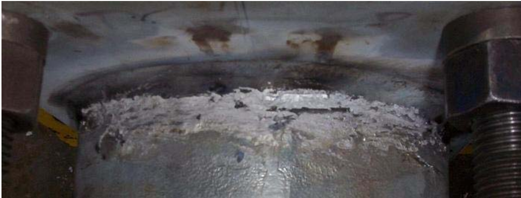
Figure 6: Mast Arm TXuCLGP After 101,865 Cycles
