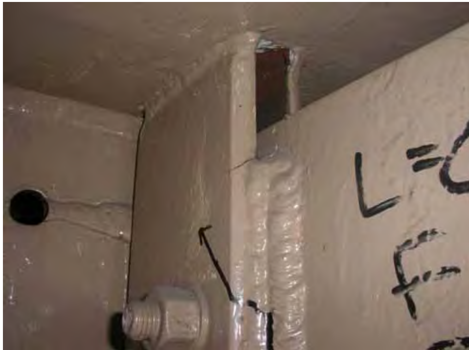
Figure 1.9: Crack at Weld Connecting Retrofit Stiffener to Existing Stiffener
