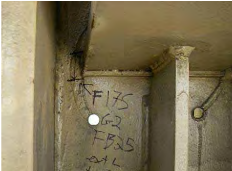
Figure 1.3: Cracked Weld Repair in Gap between Bearing Stiffener and Bottom Flange of Floor Beam
