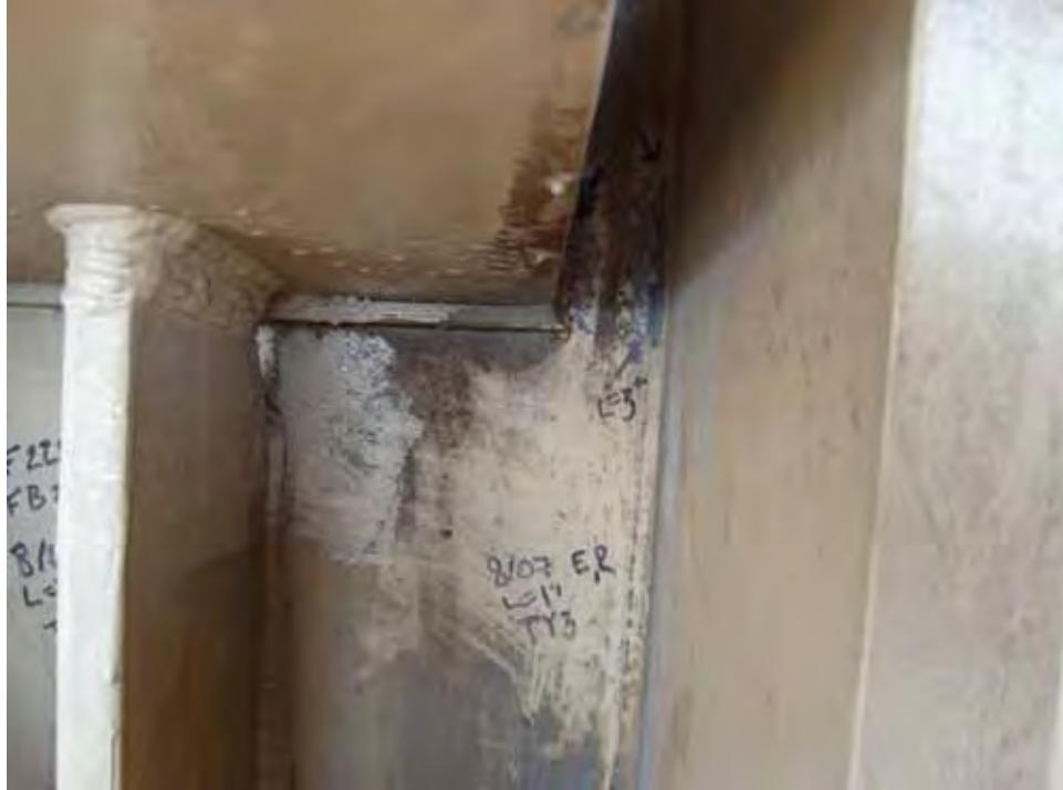
Figure 1.10: Cracks between Bearing Stiffener and Bottom Flange of Floor Beam
