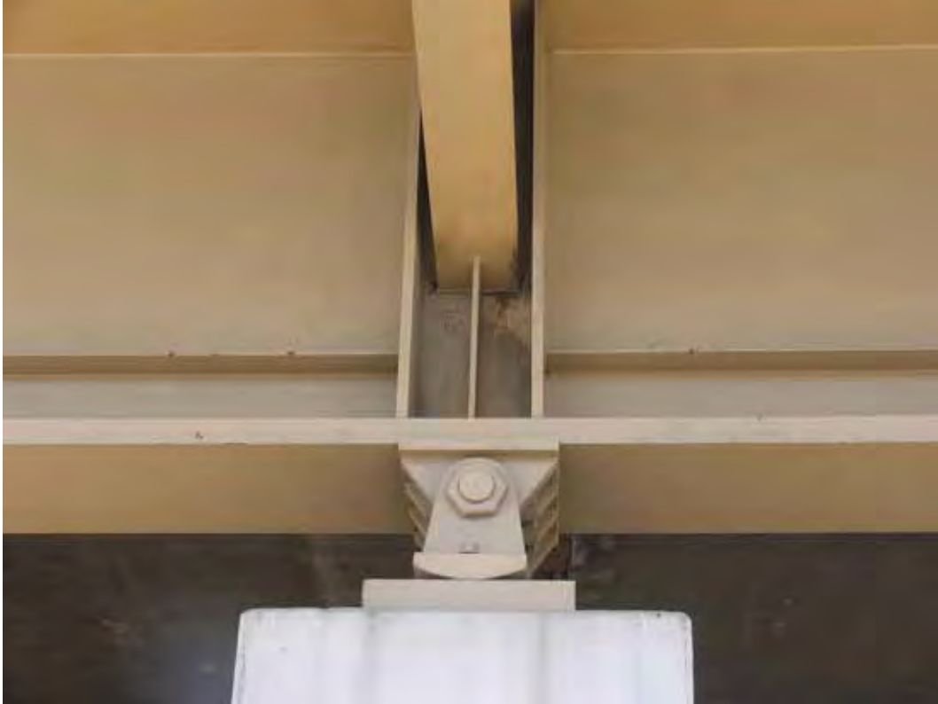
Figure 1.2: Floor Beam to Girder Connection at Pier
