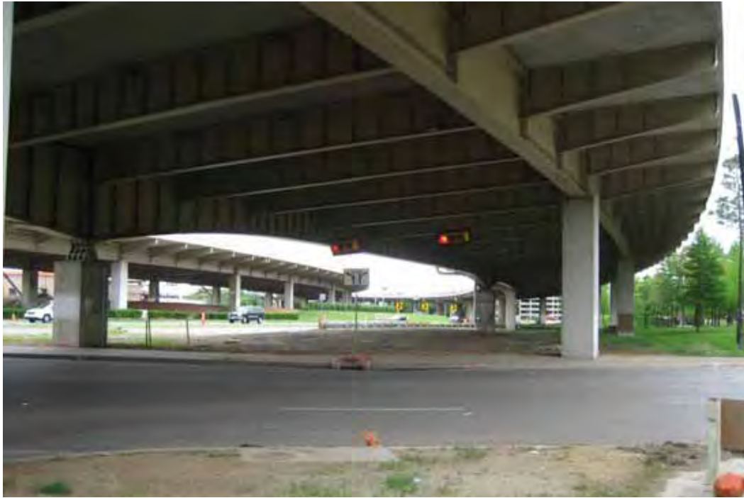
Figure 1.14: Asymmetrical Columns and Haunches of Section F17S
