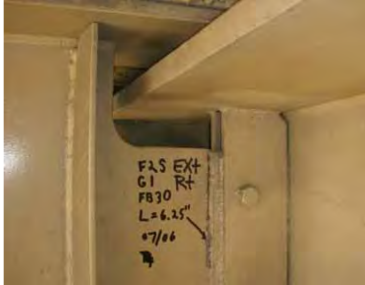
Figure 1.8: Crack at Weld Connecting Existing Stiffener to Floor Beam Web
