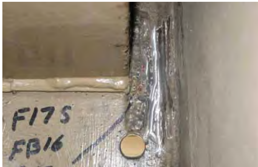
Figure 2.8: Gap between Bottom Flange of Floor Beam 16 and Bearing Stiffener
