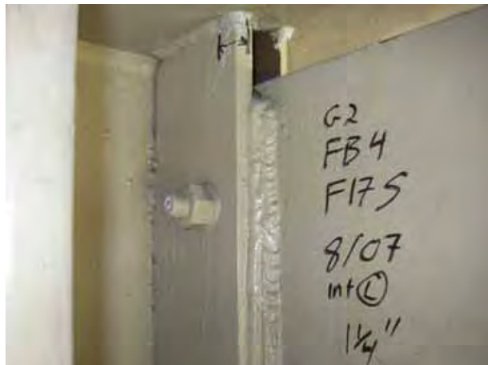
Figure 1.7: Crack at Connection of Retrofit Stiffener to Top Girder Flange
