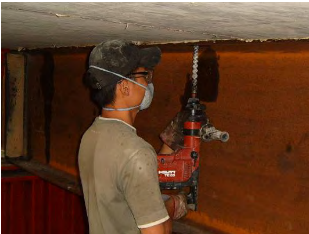
Figure B.12: Drilling into the concrete slab using a rotary hammer drill
