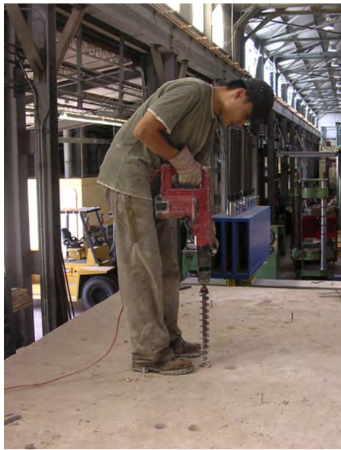
Figure B.8: Drilling into the concrete slab
