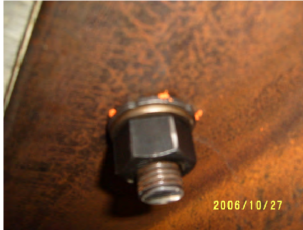
Figure B.6: Use of “Squirter” Direct Tension Indicating (SDTI) washer
