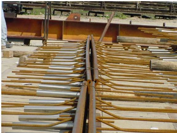
The armored joints were significantly bowed when they arrived from the steel fabricator.
