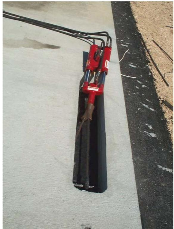
A monostrand stressing ram is used to tension the entire tendon by pulling on one strand while reacting against the other strand
