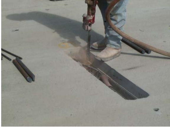
Holes are drilled into the base material at each stressing pocket for the mid-slab anchor
