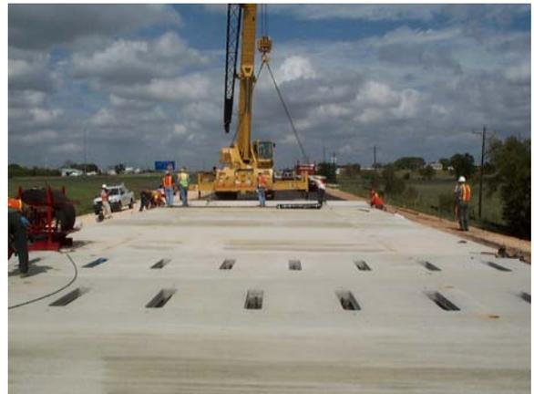
A full section of panels (between expansion joints) were placed in 6–8 hours
