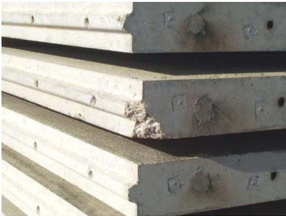
Corner breaks occurred when removing some of the panels from the forms.
