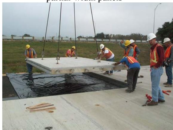
Placement of a partial-width panel over the polyethylene sheeting
