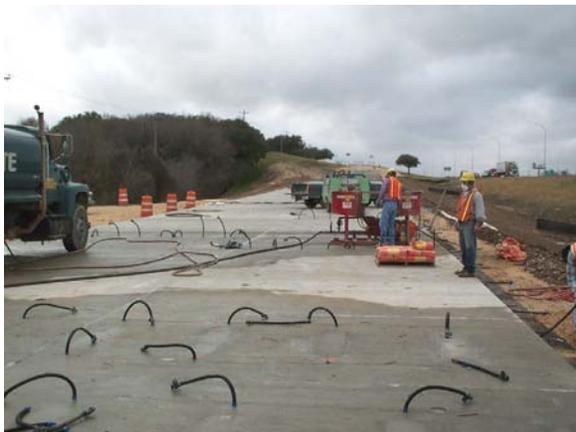
The tendons are grouted by pumping grout into the inlets/vents along the slab
