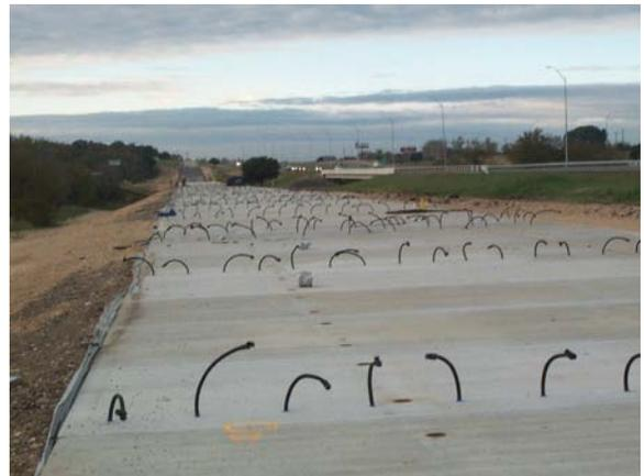
Grout tubes are attached to each inlet/vent for tendon grouting
