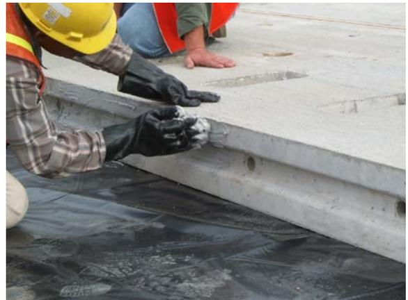
Application of segmental bridge epoxy to the panel keyways
