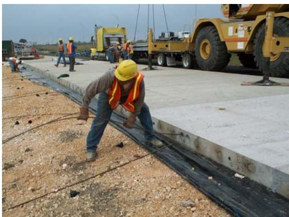
After placement of a pair of partial-width panels, the transverse post-tensioning strands were fed into the ducts.
