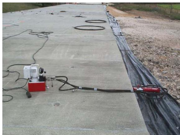
The transverse post-tensioning tendons were stressed with a monostrand stressing ram at the edge of the pavement.
