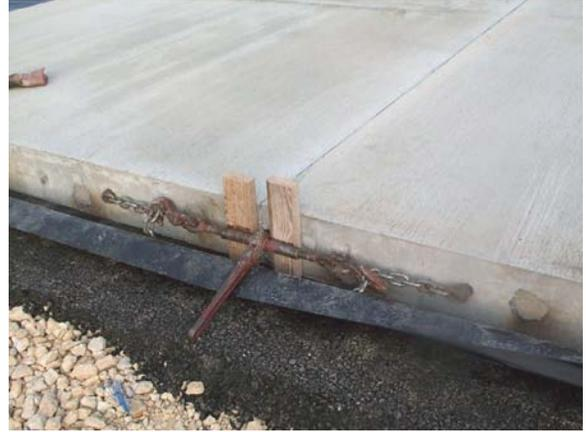
The come-alongs were used to hold the joints between panels closed as subsequent panels were placed.
