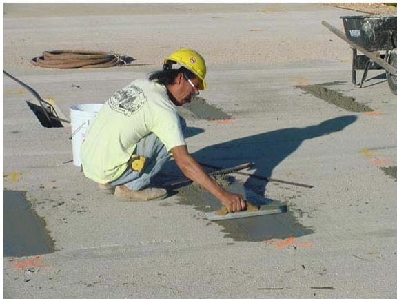
The stressing pockets and access pockets are filled prior to grouting the tendons
