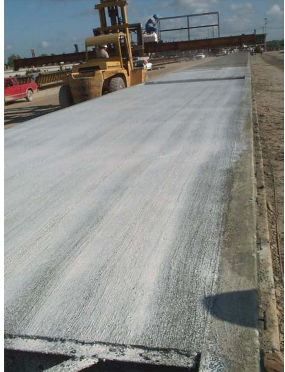
Application of two coats of curing compound to a finished set of panels
