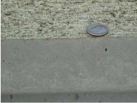
Typical mid-panel crack which occurred overnight on many of the 36 ft panels
