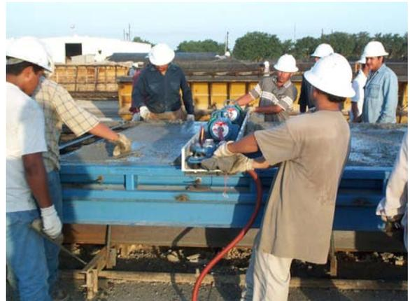
Vibratory screed used to create a flat top surface on the panels
