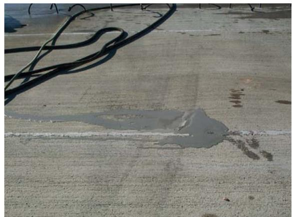
Grout leakage onto the top of the slab at the panel joints
