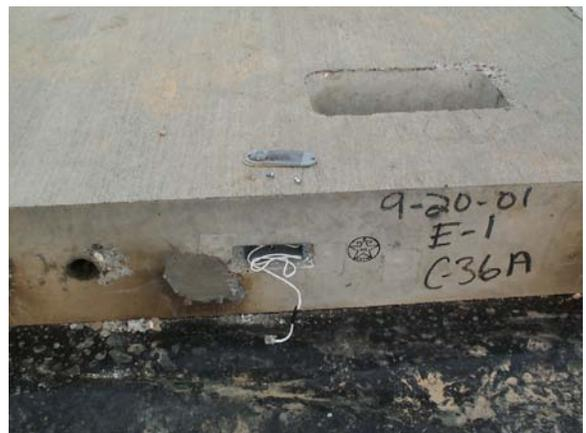
Removable covers provide access to the temperature instrumentation at the edge of the slab
