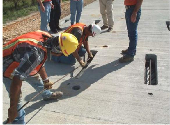
The longitudinal post-tensioning strands are fed into the ducts at the Central Stressing Panels and fed by hand to the anchors in the Joint Panels.
