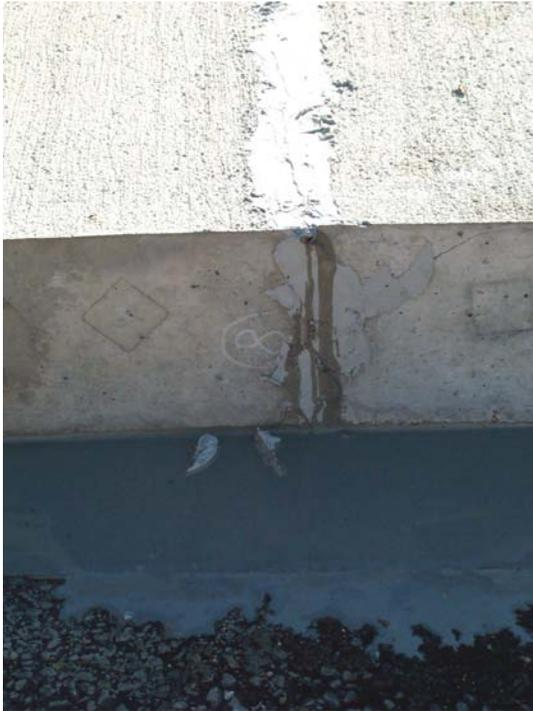
Grout leakage from the ends of the panel joints
