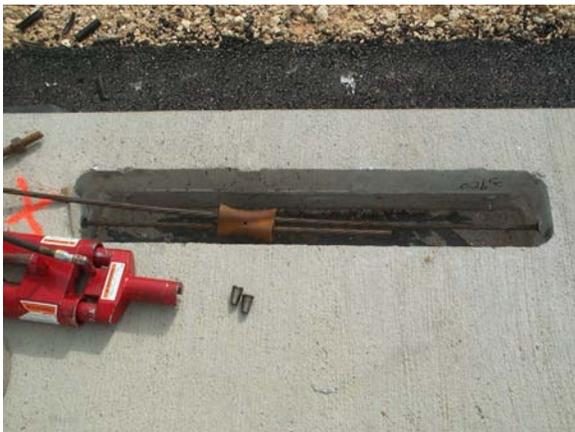
The strands coming into the stressing pockets from either end of the slab are coupled together with a ring anchor
