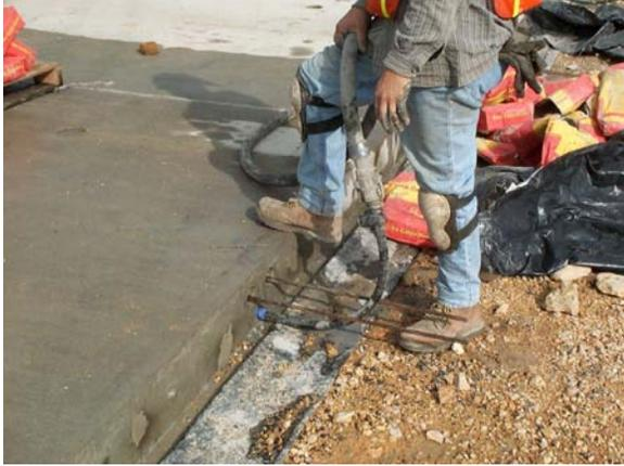
After stressing, the transverse post-tensioning tendons were grouted.
