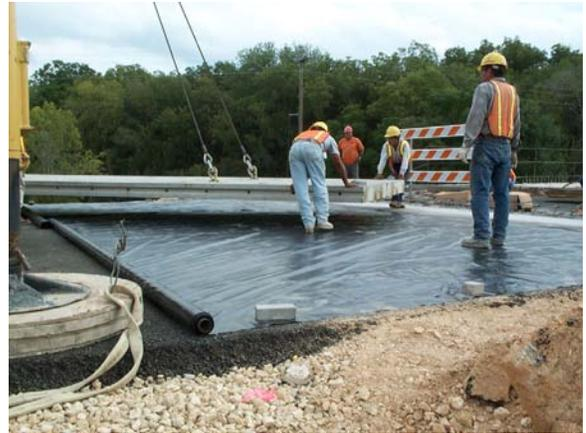
Placement of a joint panel over the polyethylene sheeting
