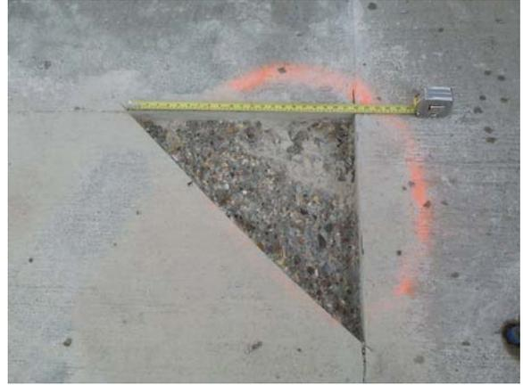
Typical on-site repair to a corner crack in a partial-width panel at the joint between 16-ft and 20-ft panels
