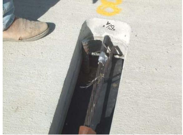
A #7 deformed bar is grouted in the hole to provide the mid-slab anchor
