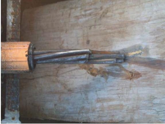
When pushing the strands through the ducts, some of the individual wires would push back, leaving only 4 – 5 wires to go into the anchor.
