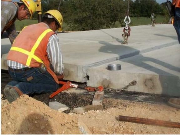
Come-alongs linked between the edge sleeves were used to pull the panels together as they were lowered into place
