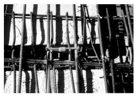
Figure 4.10 Instrumentation tied into cast-in-place deck reinforcement
