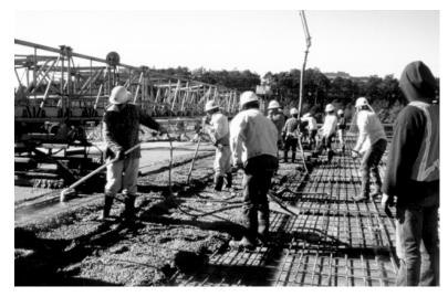
Figure 4.11 Casting operations for the bridge decks
