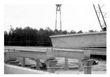
Figure 4.7 U-beam being erected in the bridge
