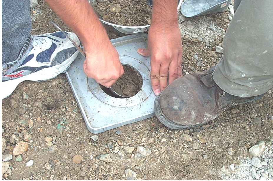
Figure 2.11 Excavation of hole for rubber balloon test.
