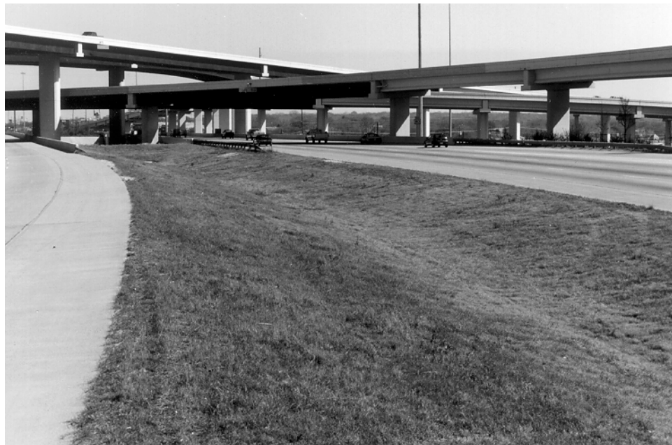
Figure 2.2 Vegetated Buffer Strip at US 183 Site
