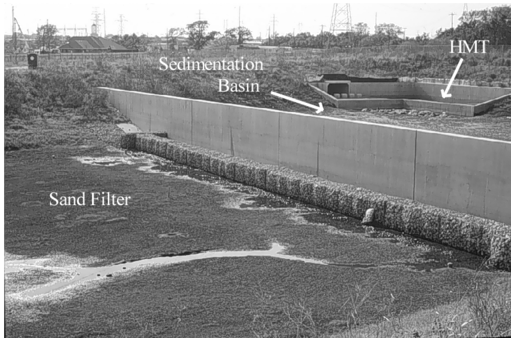
Figure 3.2 Seton Pond Sedimentation/Filtration Facility
