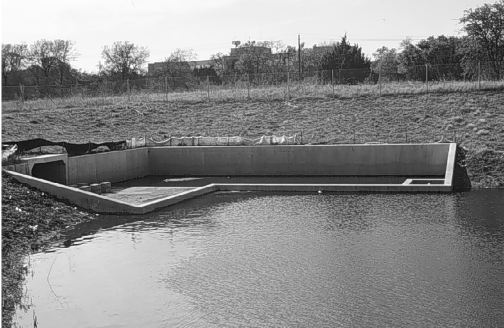
Figure 3-5 Hazardous Materials Trap
