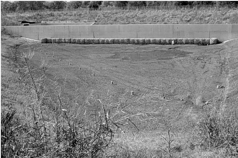
Figure 3-6 Seton Pond Sand Filter
