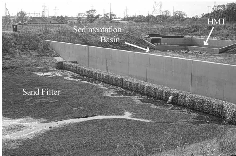
Figure 3-2 Seton Pond Sedimentation/Filtration Facility
