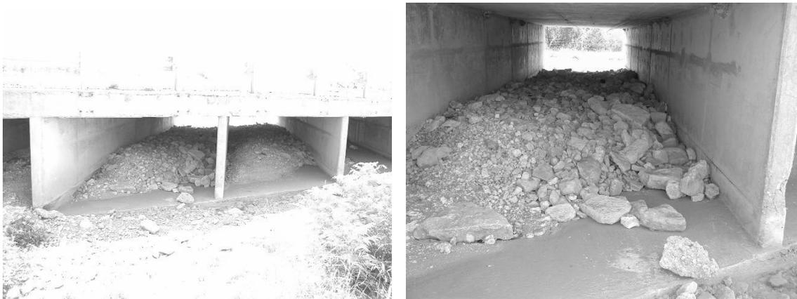
*Figure 1.4 Sediment accumulation within the culvert boxes*
