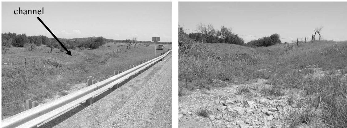
*Figure 1.2 Upstream view from culvert showing poorly defined channel*
