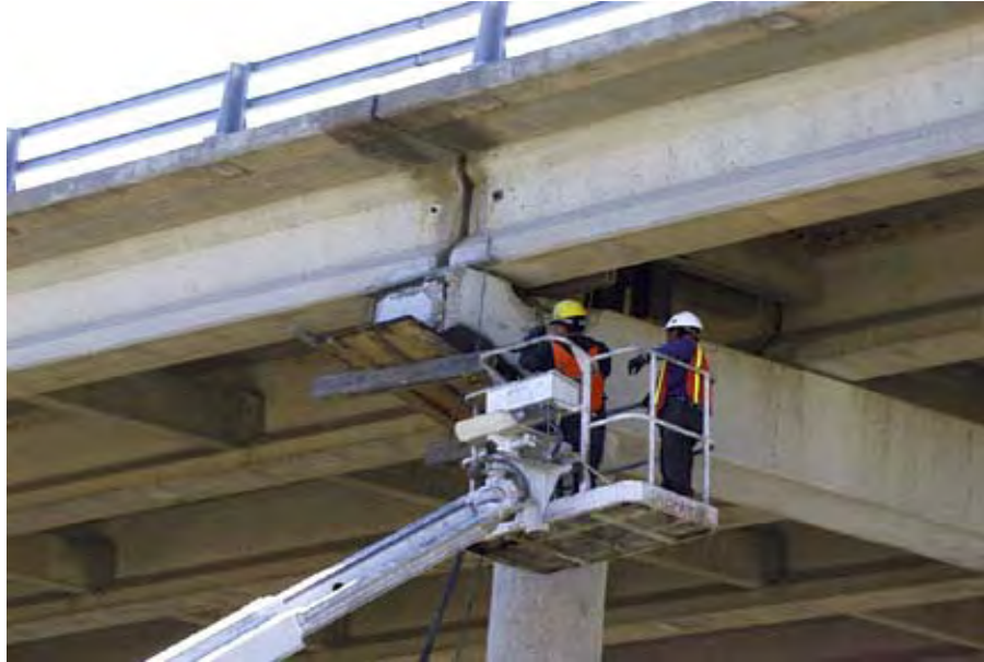
Figure 5.4 Application of Shotpatch® 21F to Structure #3
