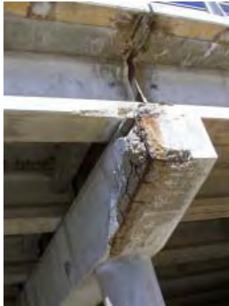
Figure 3.1 Endcap delamination
