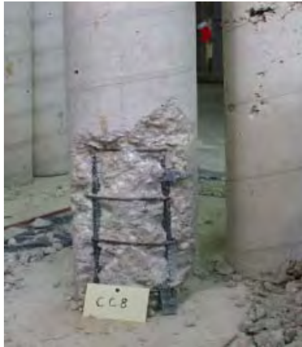
Figure 4.8 Concrete removed prior to repair
