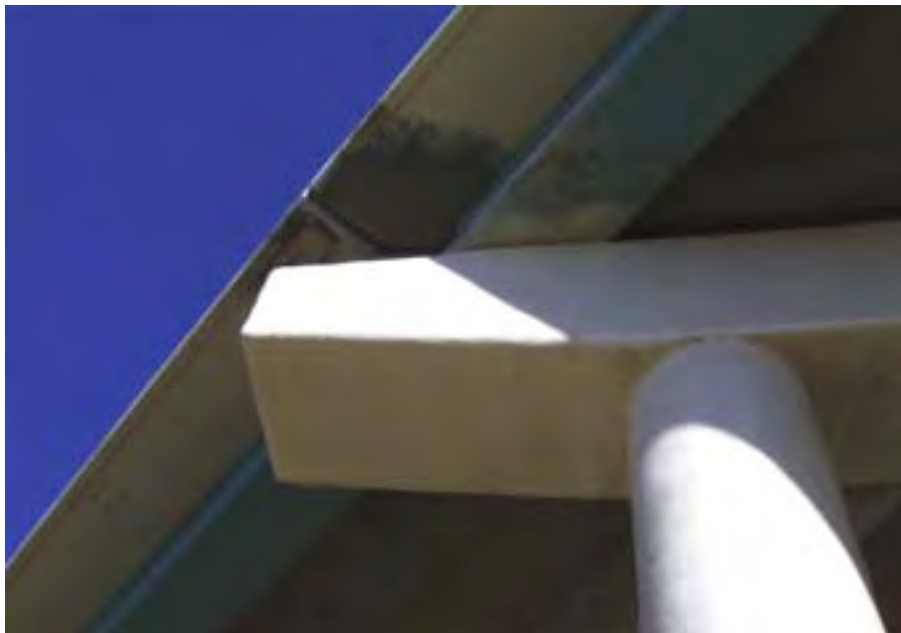
Figure 5.9 Wrapped and painted endcap on Structure #2
