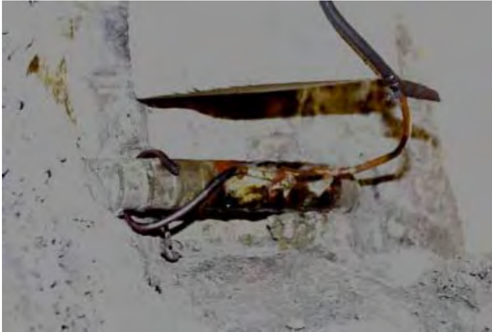
Figure 5.20 Typical silver soldered electrical connection
