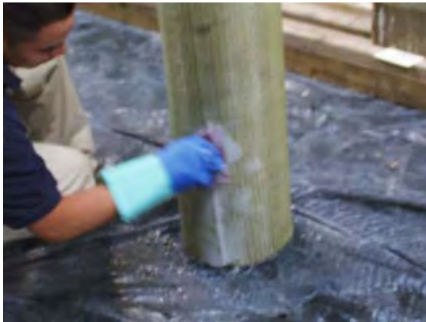
Figure 4.17 Sealing joints of column wrap
