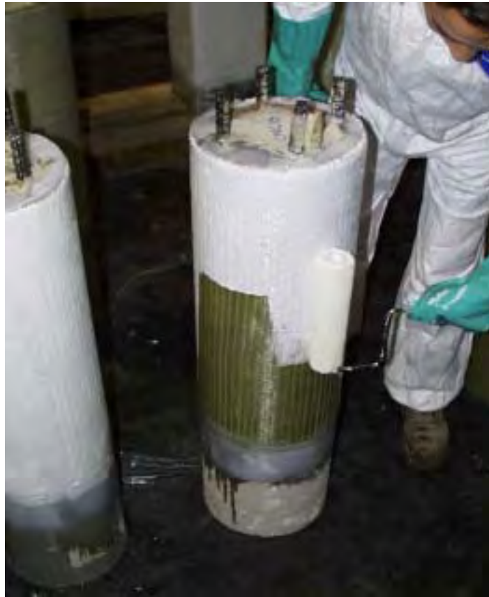
Figure 4.18 Painting wrapped column
