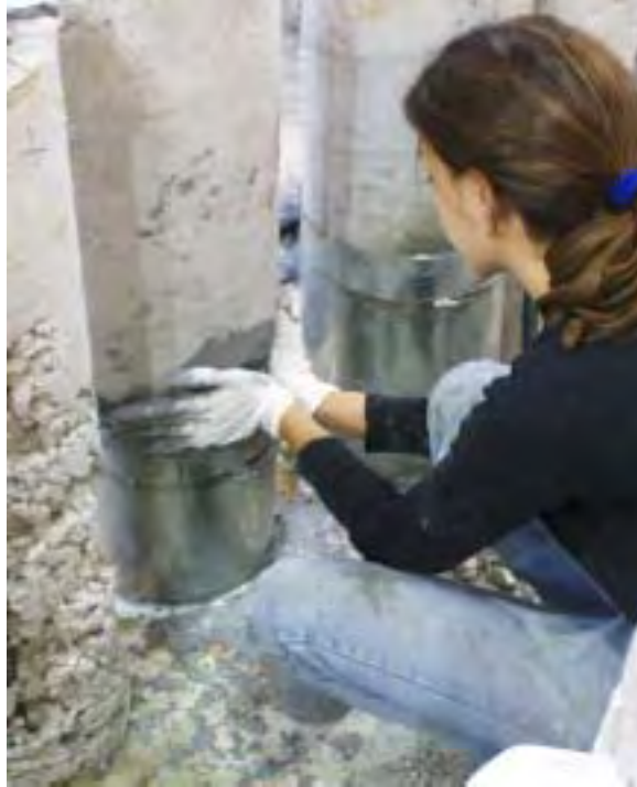
Figure 4.11 Drypacking procedure
