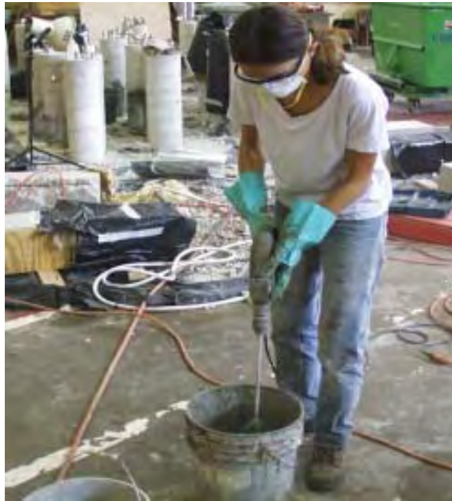
Figure 4.9 Mixing repair materials
