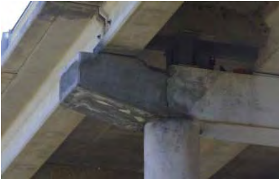
Figure 5.5 Endcap repair material on Structure #3
