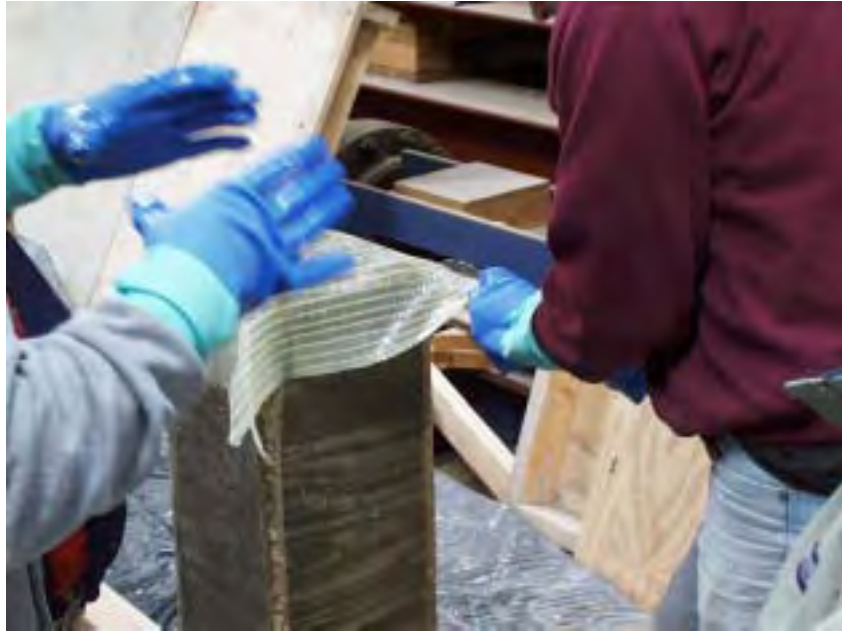
Figure 4.14 Wrapping beam end
