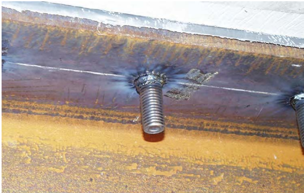
Figure 6.64 Close up view of the threaded stud
