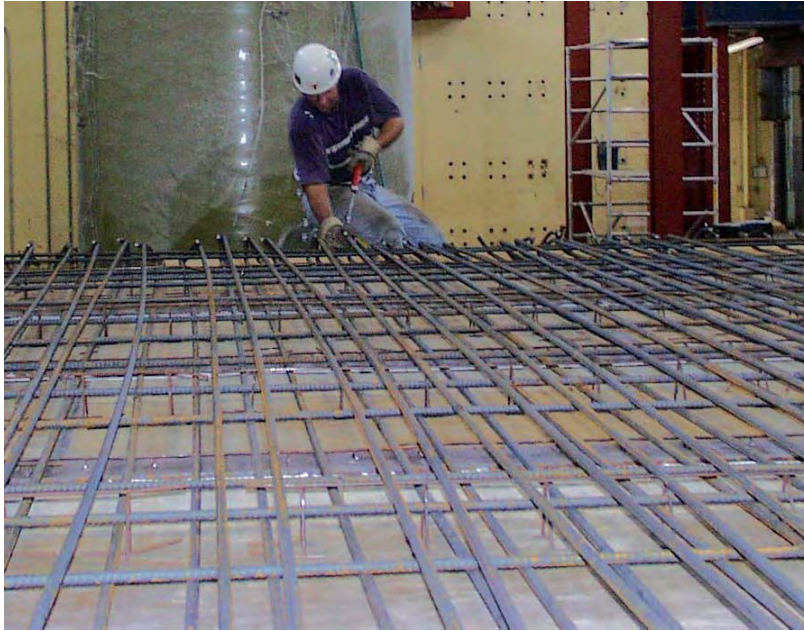
Figure 6.11 Reinforcing bar placement in slab
