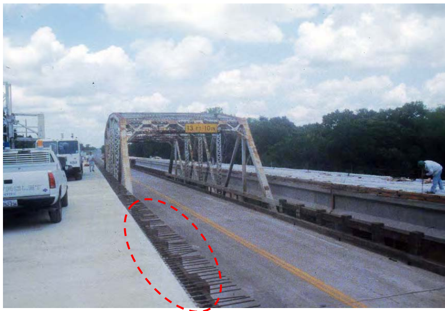
Figure 5.3 Detail showing connecting rebar
