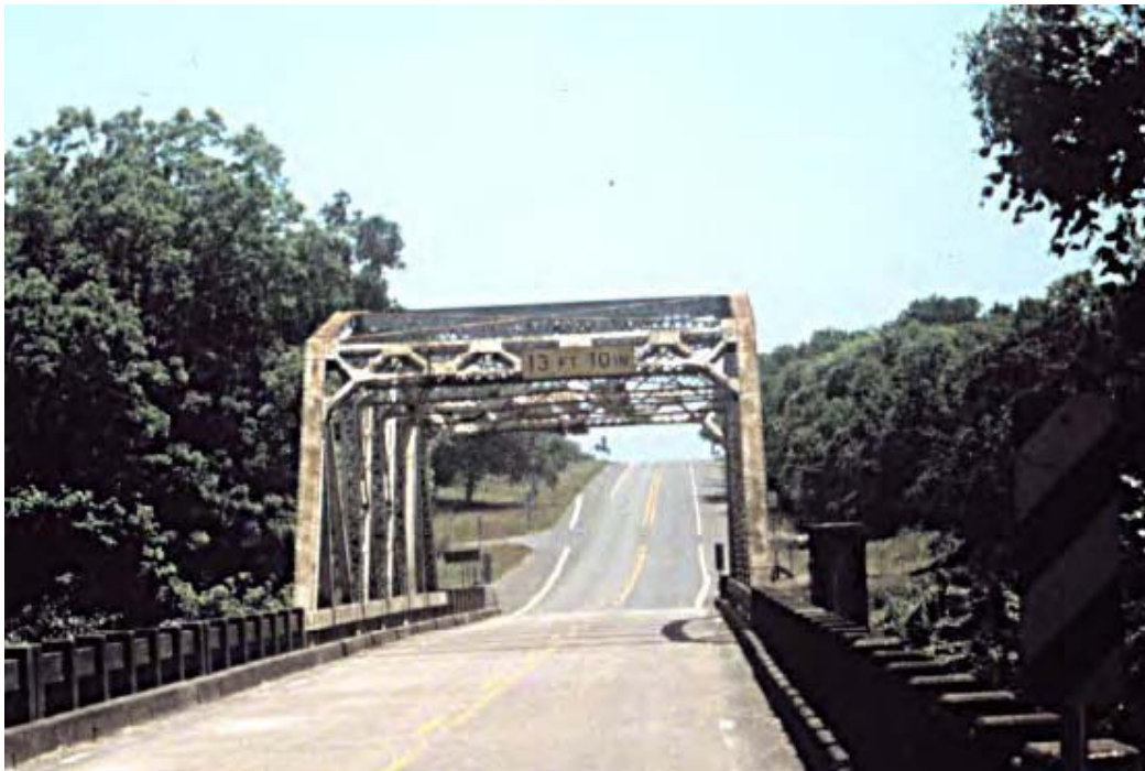
Figure 5.1 Parker truss bridge in Goliad, Texas
