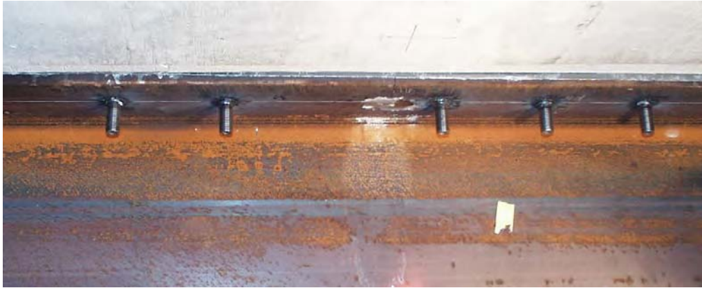
Figure 6.63 Threaded studs welded to the inside top flange of the transverse beam
