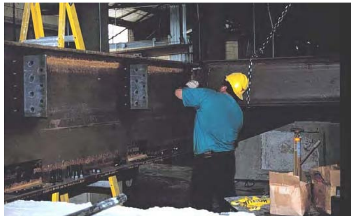
Figure 6.5 Connecting of longitudinal stringer to transverse beam
