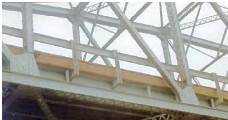
Figure 2.11 Angle attachments of railing to longitudinal stringers
