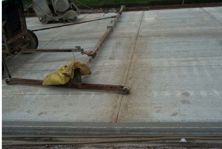
Figure 4.14: Early entry sawing
