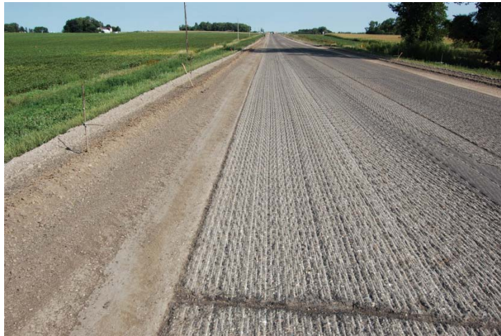
Figure 4.3: Milled existing asphalt pavement
