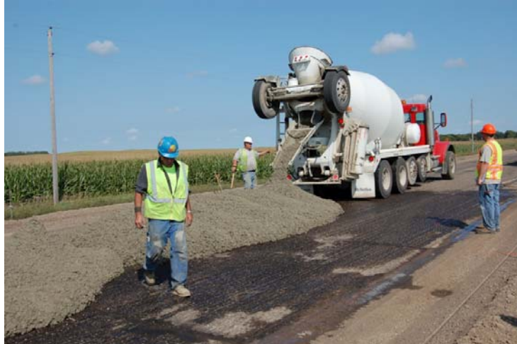
Figure 4.6: Wetted surface and dried surface
