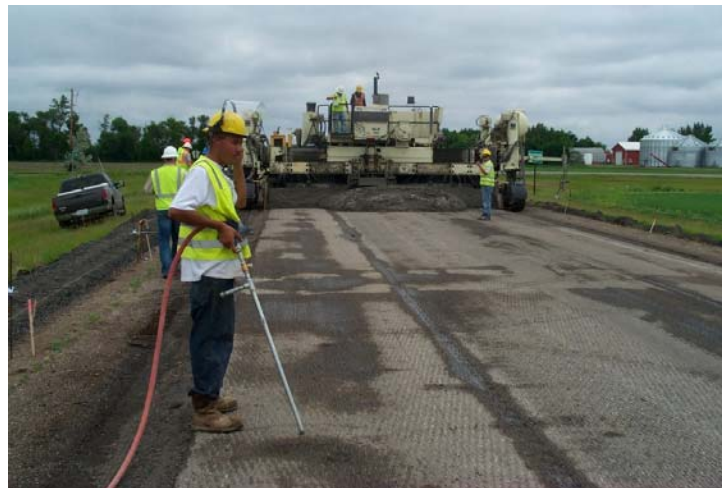
Figure 4.5: Use of an air hose to clean the surface and spread pooled water just ahead of the paver
