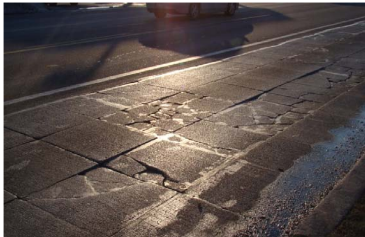
Figure 2.6: Failed joints in wheel path
