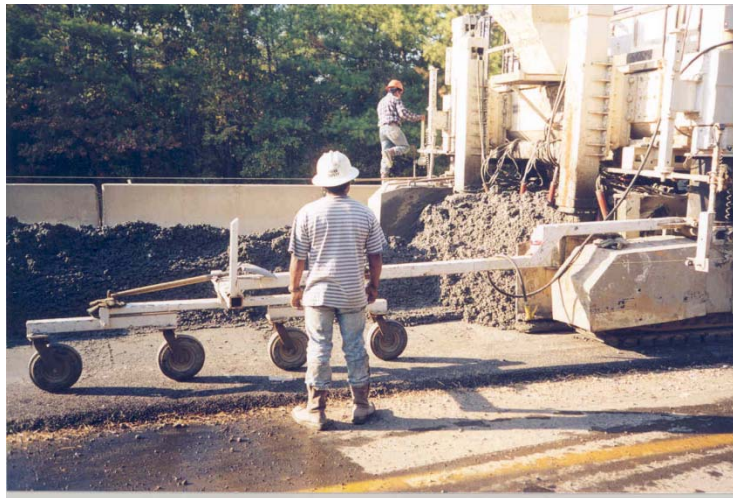
Figure 4.9: Existing pavement, 2-in. thick asphalt separation layer, and concrete overlay placement
