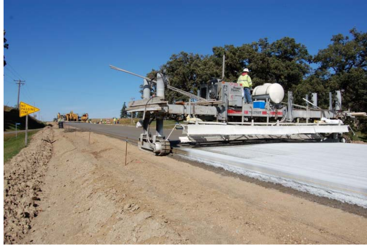
Figure 4.13: Curing compound being promptly applied following paving operation
