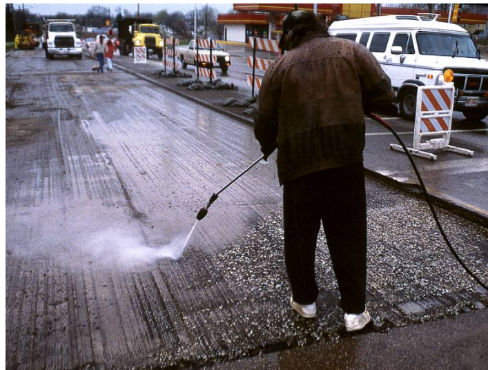
Figure 2.5: Cleaning the surface with hydrocleaning equipment
