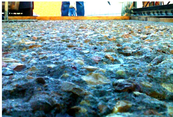
Figure 4.4: A shot blasted existing concrete pavement
