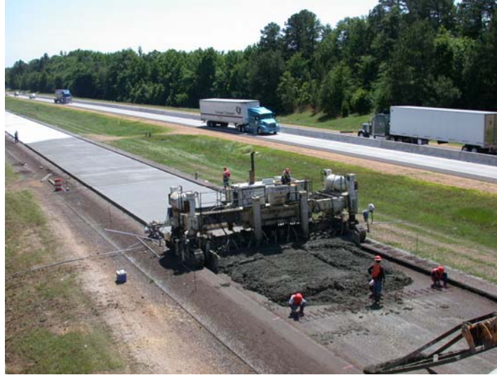
Figure 2.7: Prompt curing following the paver
