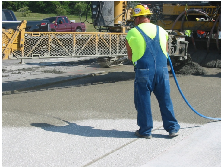
Figure 4.11: Grout, as a bonding agent, being placed evenly just ahead of paver
