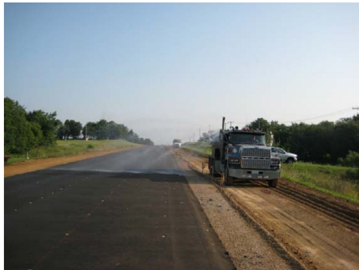
Figure 2.4: Cooling down the prepared surface before placement
