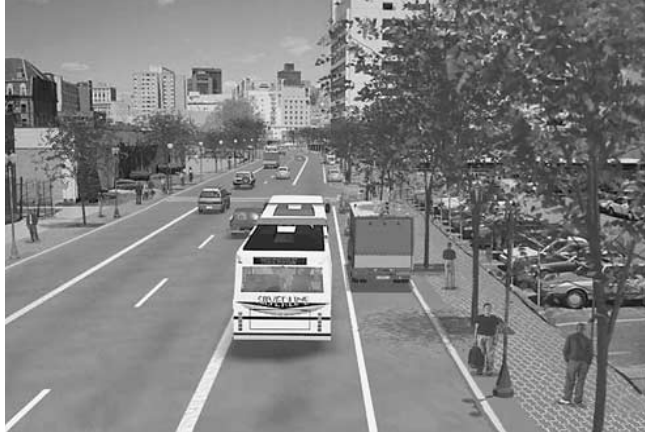
Figure 7.5: Concurrent Flow Interior Bus Lane—Silver Line, Boston (Levinson et al. 2003)
