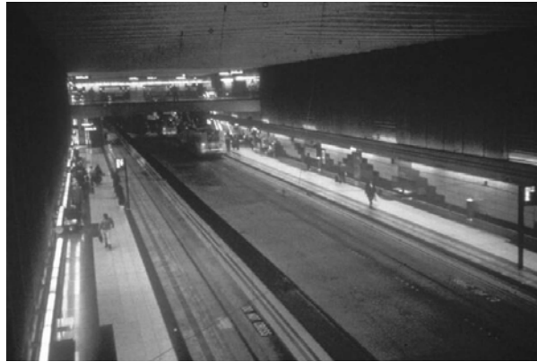
Figure 7.1: The Bus Tunnel in Seattle (1)
