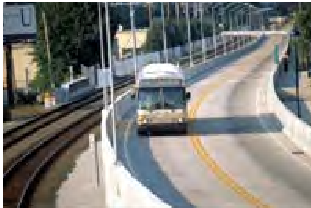
Figure 7.2: Grade-separated Busway, Pittsburgh (2)
