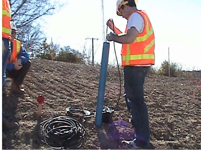
Figure 9.6: Taking Inclinometer Readings
