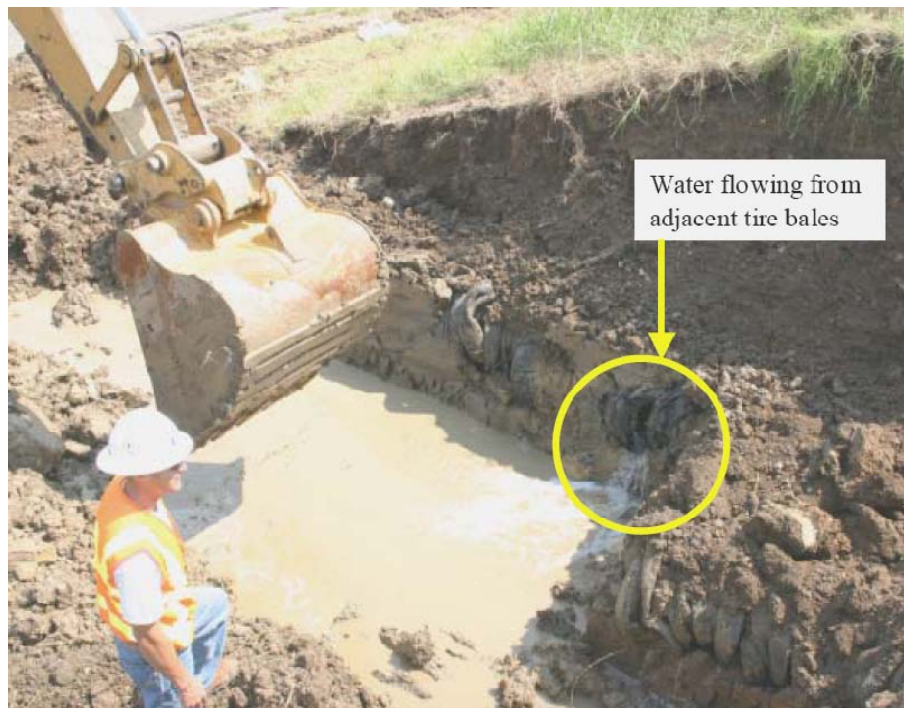
Figure 2.18: Water Flow from the Tire Bale Reinforcement Layers (LaRocque 2005)
