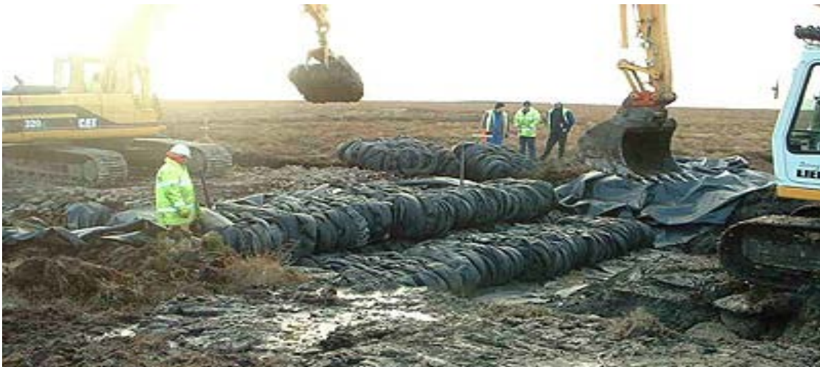
Figure 2.14: Lightweight Tire Bale Road Construction ( www.angloenvironmental.com/tyre_blocks_anglo.php )
