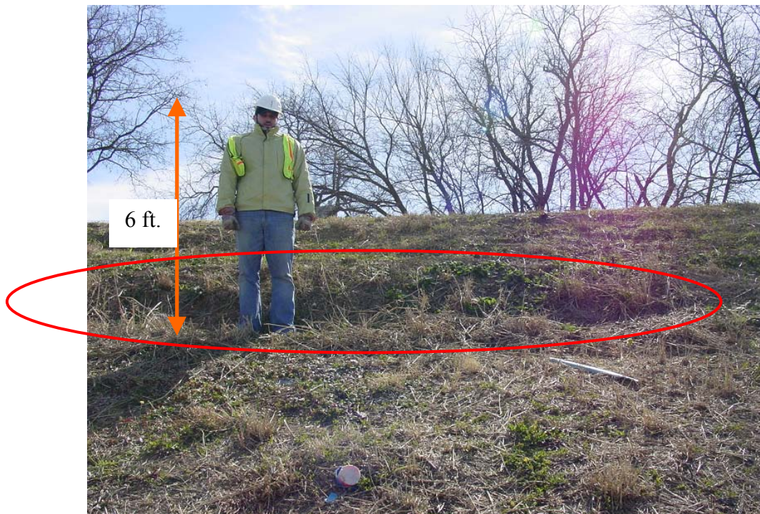
Figure 9.12: Soil Slump Observed at the Upper East Corner of the Tire Bale Slope
