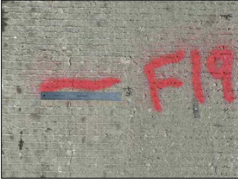
Figure 3.45: 0.030 in. Crack
