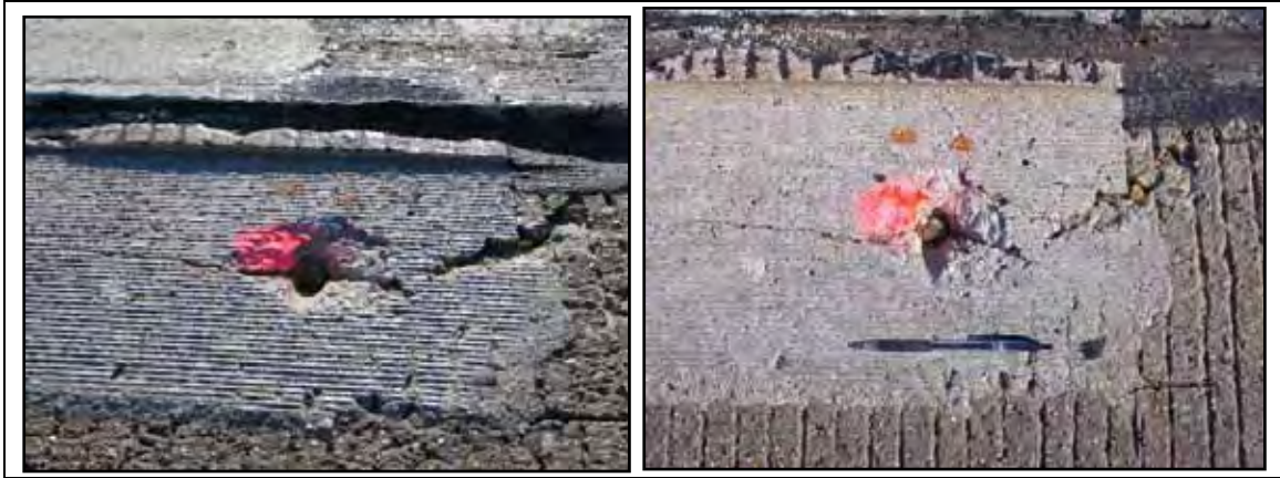
Figure 4.68: Cross Stitching Distress on US 59
