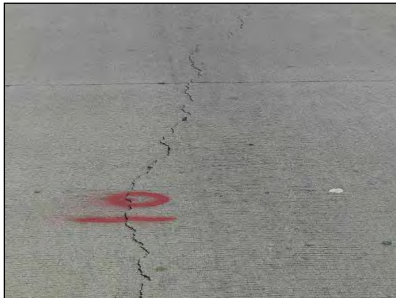
Figure 3.26: Longitudinal Cracking (2)
