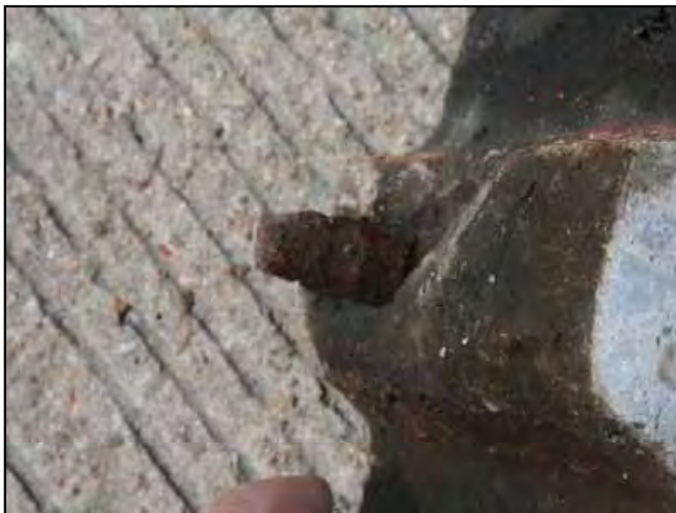
Figure 6.10: Slab 13 Corroded tie bar in keyed joint
