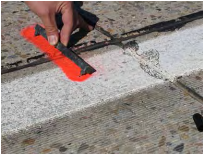
Figure 3.4: Installation of Joint Width Monitoring Pins
