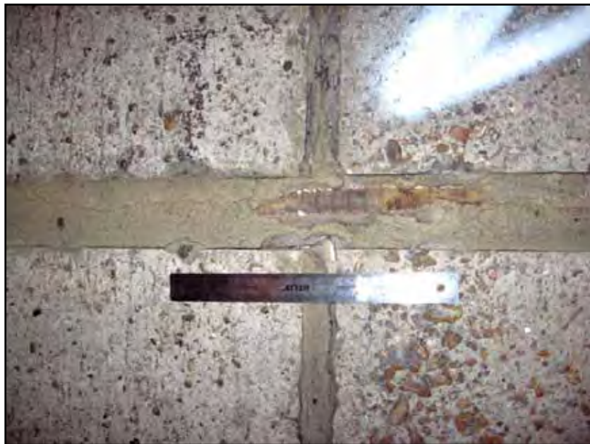
Figure 3.20: Staple Corrosion
