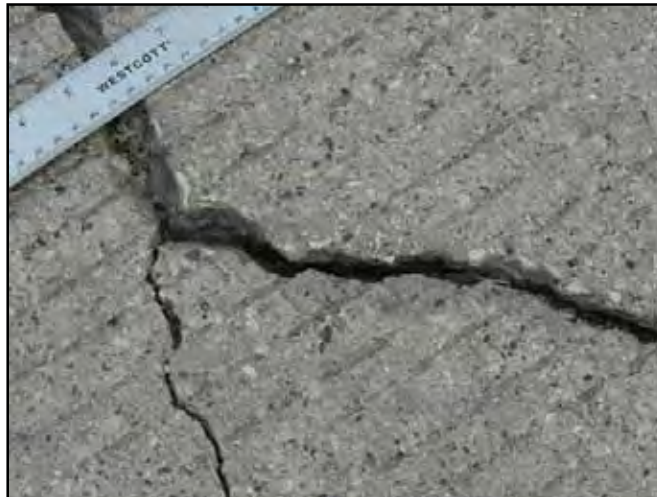
Figure 3.28: Wide Crack with Faulting
