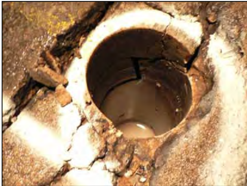
Figure 4.79: EL Paso Core Hole with Longitudinal Cracking
