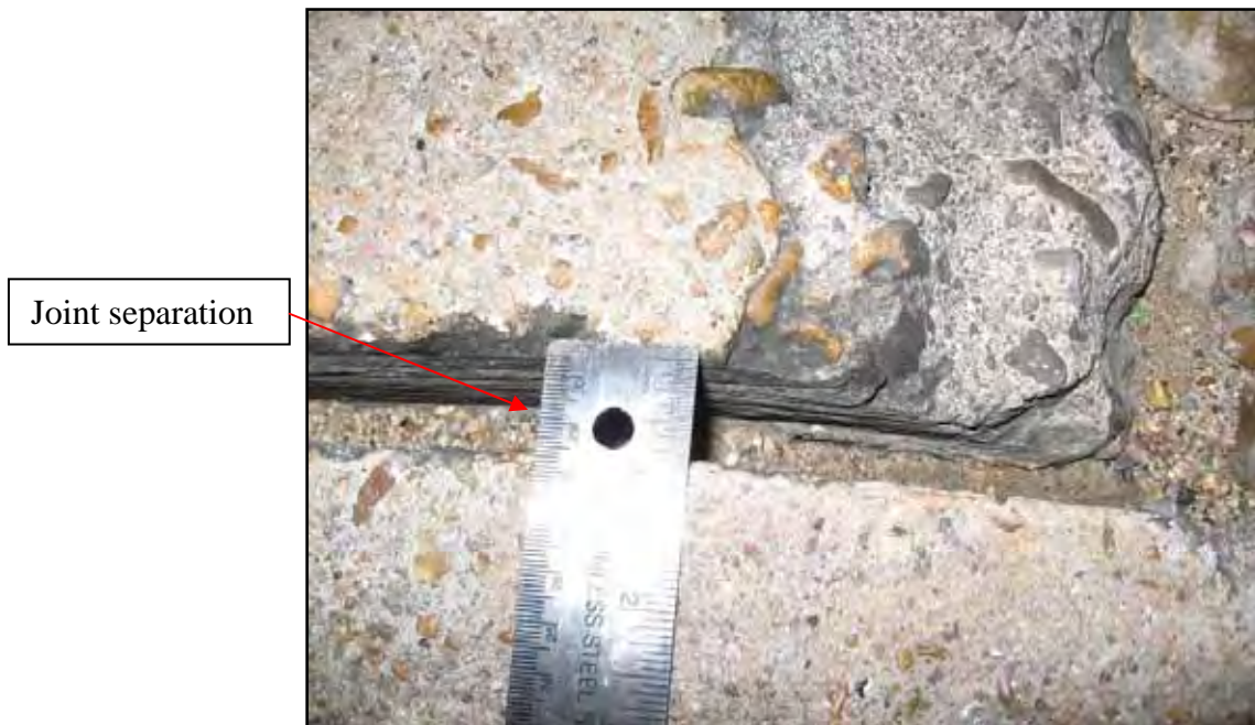
Figure 4.90: Houston US 290 Joint Separation
