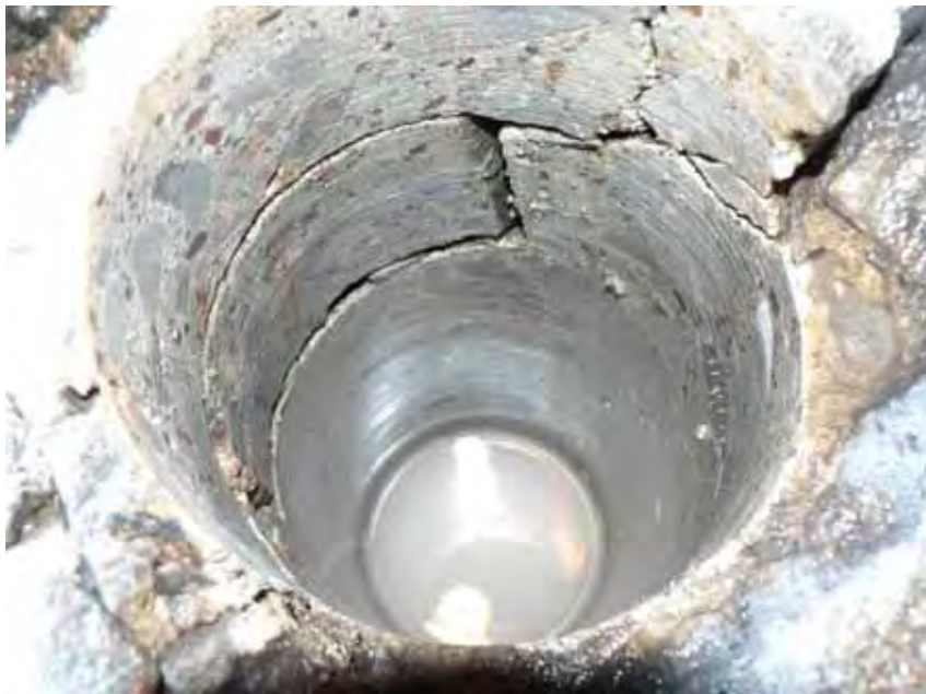
Figure 3.80: Core Hole Through Joint (2)
