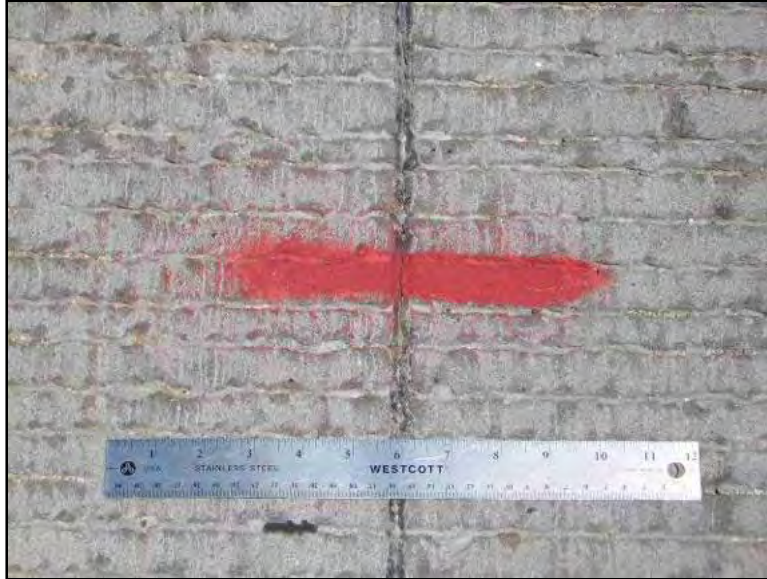
Figure 3.53: Longitudinal Warping Joint
