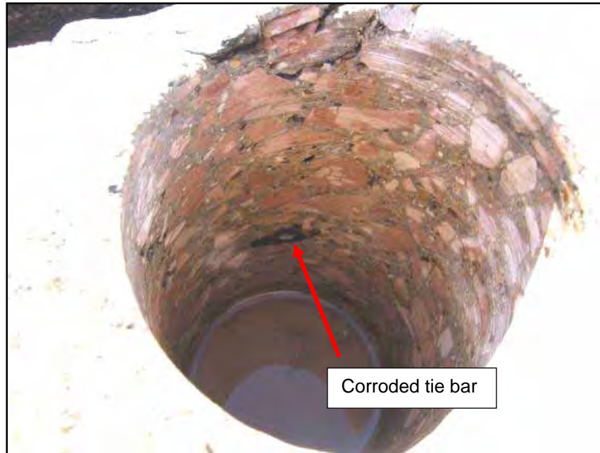
Figure 3.72: Core Hole Over Tie Bar
