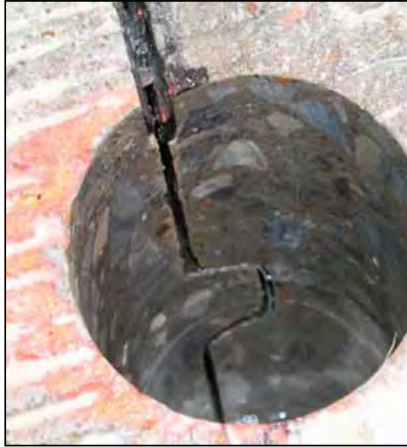
Figure 6.9: Slab 13 Keyed joint
