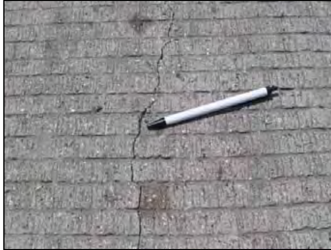
Figure 3.27: Narrow Crack
