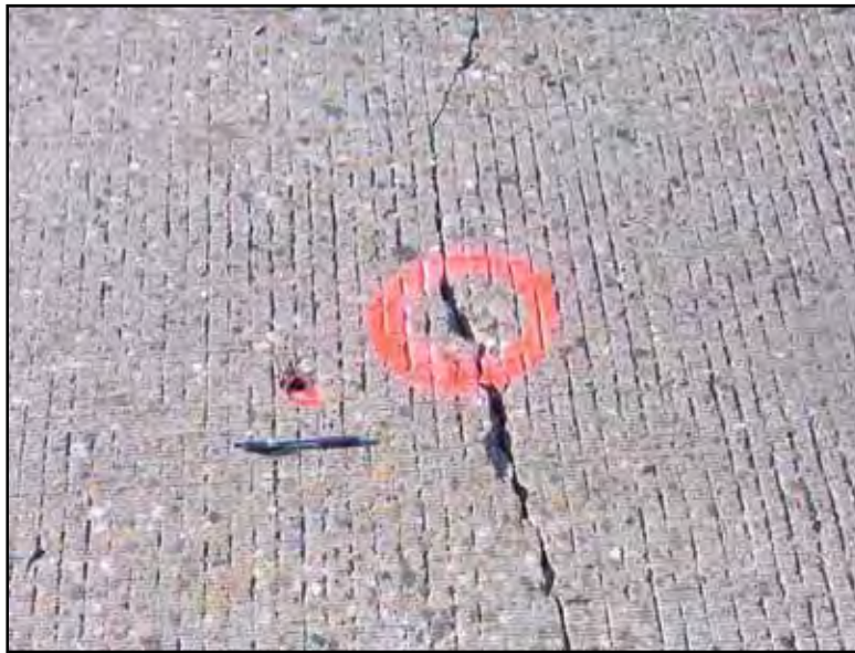
Figure 3.6: Transverse Slab Crack in Area Two
