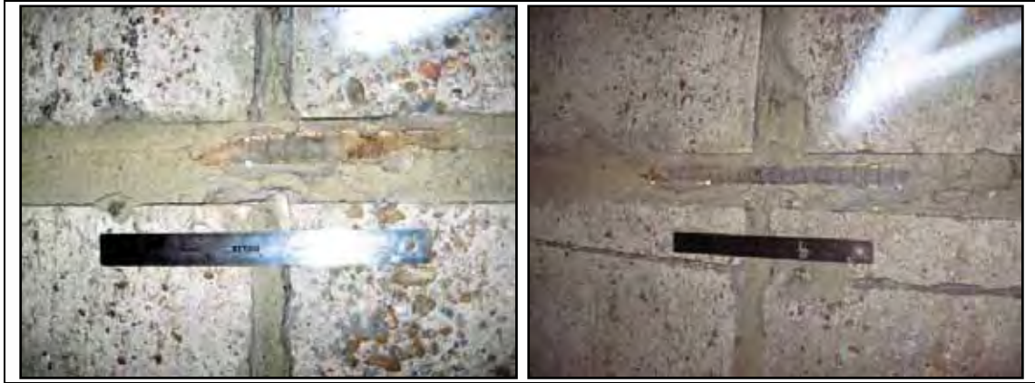
Figure 4.69: Deterioration of Stapling on US 290
