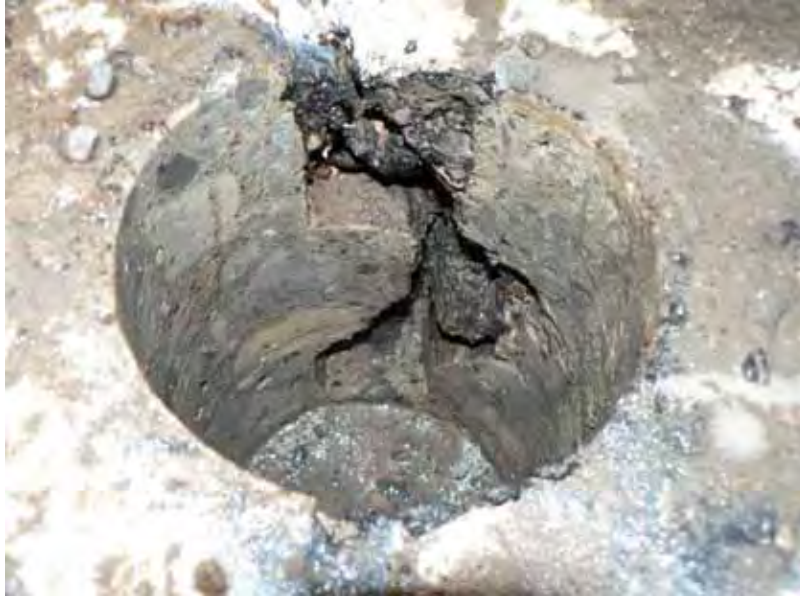
Figure 3.79: Core hole through joint (1)
