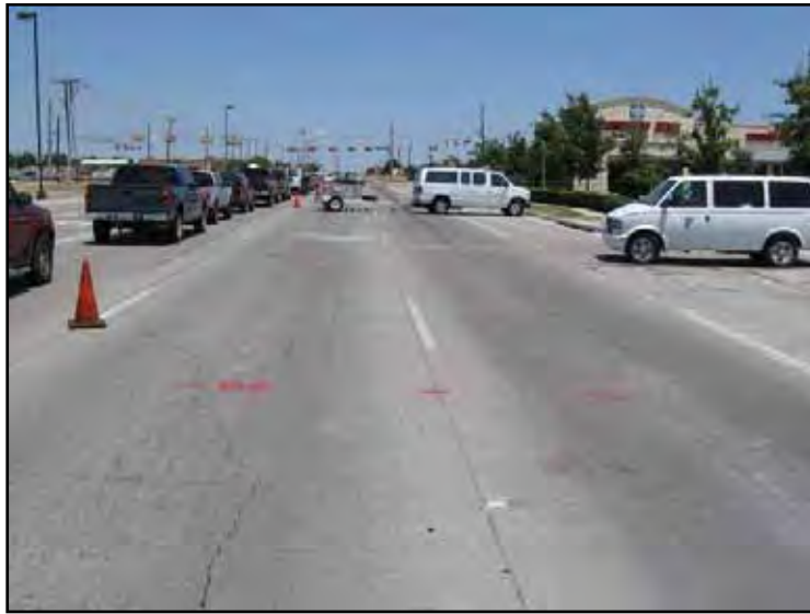
Figure 3.40: Longitudinal Cracking (1)
