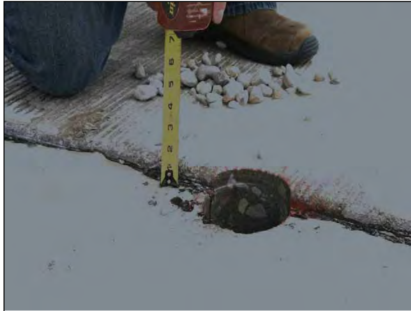
Figure 6.7: Faulted Slab 5
