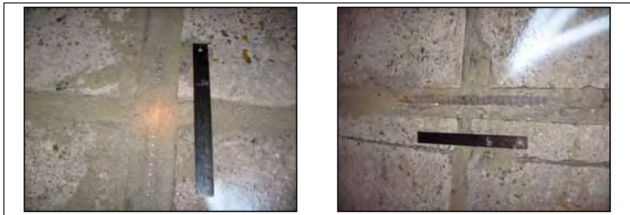
Figure 3.23: Protruding Staple Bars
