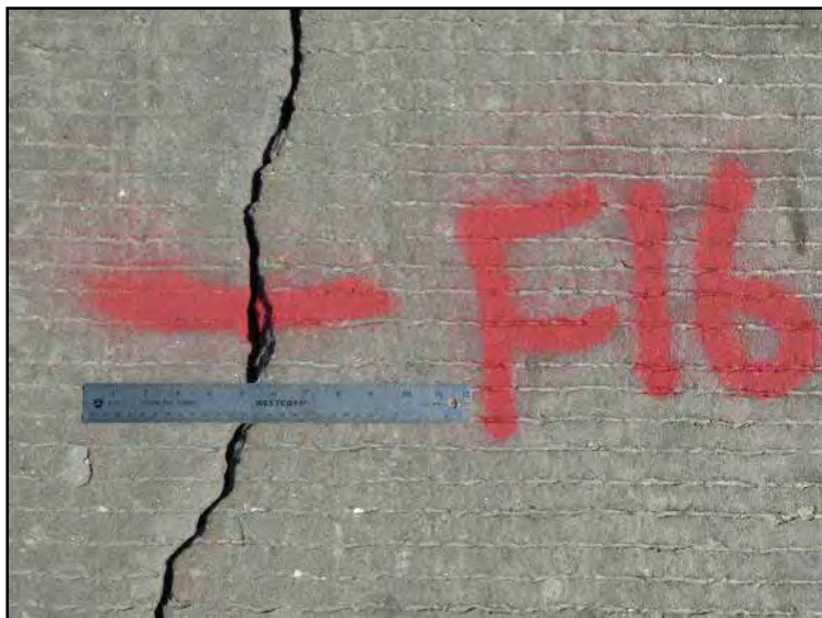
Figure 3.44: 0.625 in. Crack
