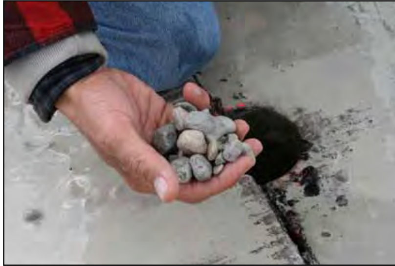
Figure 6.5: Subbase Material Resulting from Slab Pumping at Slab 5
