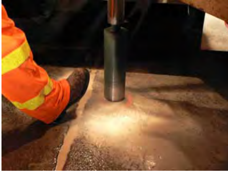
Figure 3.77: Coring Operation
