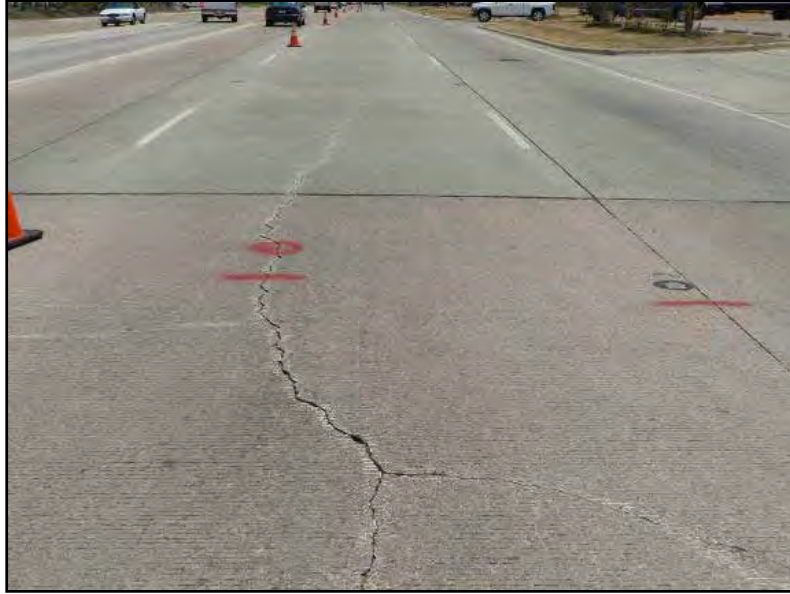
Figure 3.25: Longitudinal Cracking (1)
