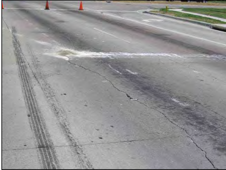
Figure 3.41: Longitudinal Cracking (2)
