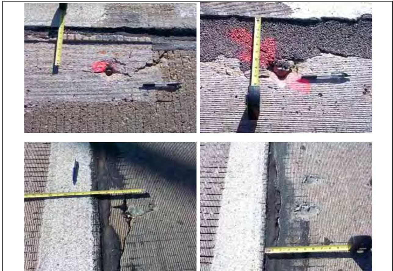
Figure 3.18: Distressed Stitching in Area Three
