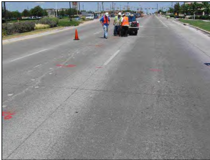
Figure 3.42: Cross-Stitch Repair (1)
