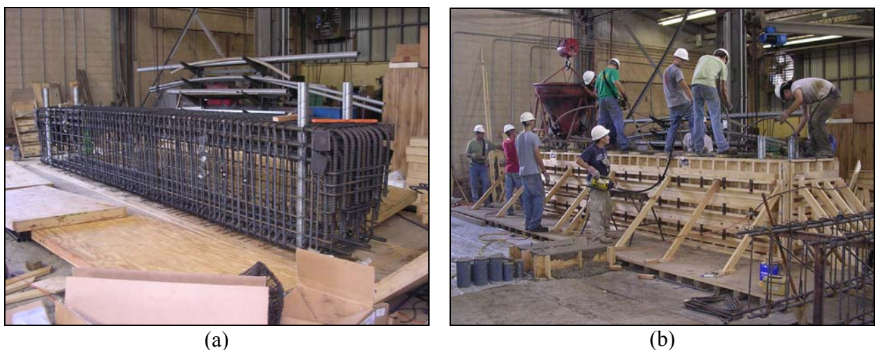
Figure 3.22: Fabrication of a 36"x48" beam: (a) tied reinforcement cage (b) placement of concrete into wooden formwork
