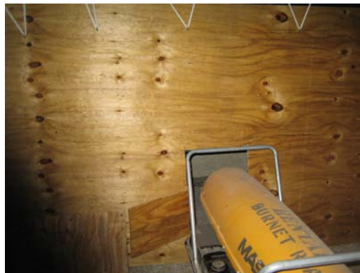
Figure 5.4: Kerosene heater used to heat tent enclosure
