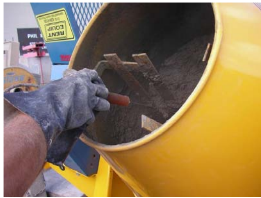
Figure 5.5: HWRA used to increase concrete fluidity
