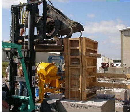
Figure 5.7: Pouring of the concrete into column forms
