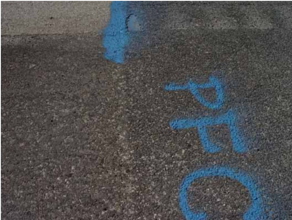
Figure 6.26: Old PFC on IH-35 in Waco, from September 2006
