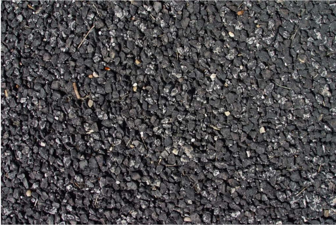
Figure 4.37: Pavement texture of IH-35 PFC in Waco
