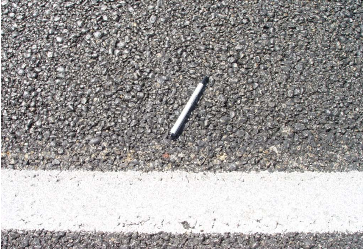
Figure 4.30: Pavement texture of SH 6 PFC in Waco
