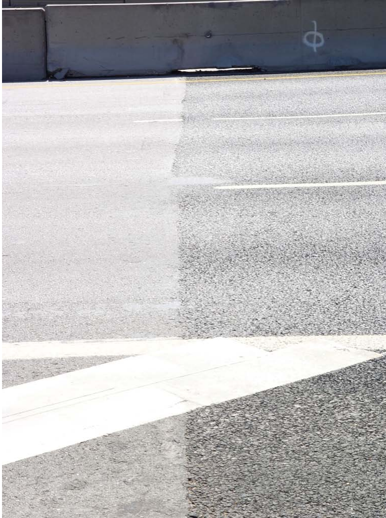
Figure 4.23: Westbound transition to new PFC overlay on IH-30 in Dallas
