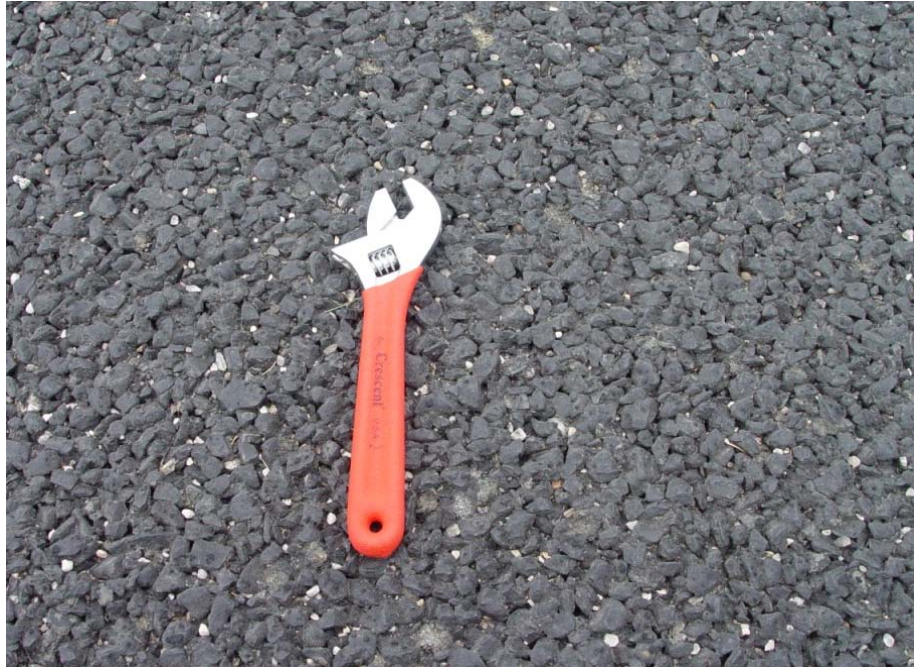
Figure 4.56: Texture of asphalt rubber PFC1 section on US 281 in San Antonio
