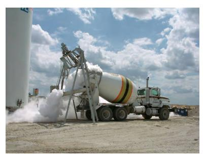
Figure 2.3 Cooling fresh concrete with liquid nitrogen
