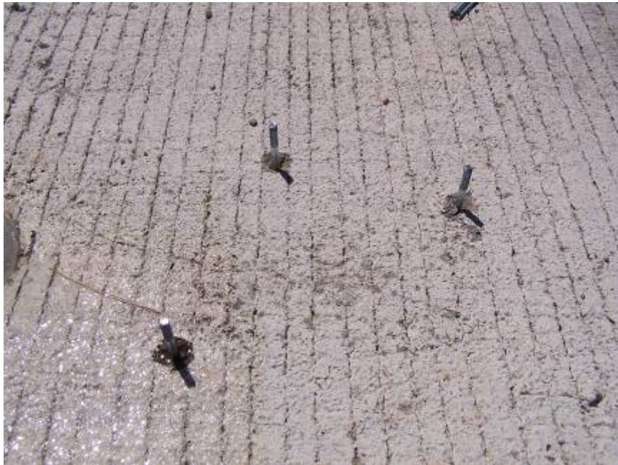
Figure 2.4: Field application of the Windsor probe system
