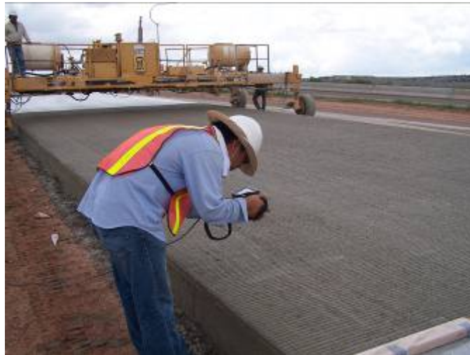
Figure 2.6: Surface temperature measurement by infrared camera
