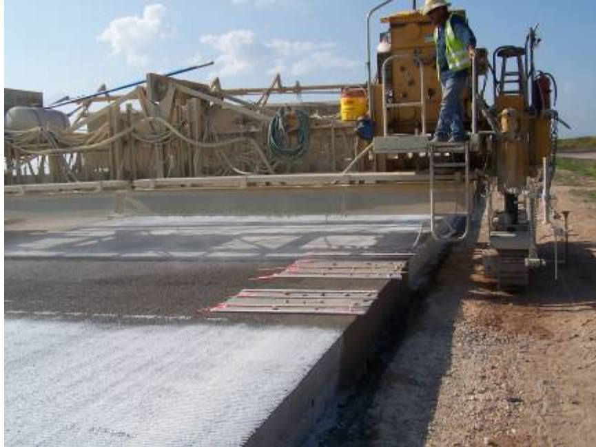
Figure 2.3: Control of application of curing compound with plastic sheet
