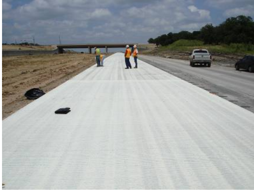
Figure 2.21: Non-uniform distribution of curing compound in the field
