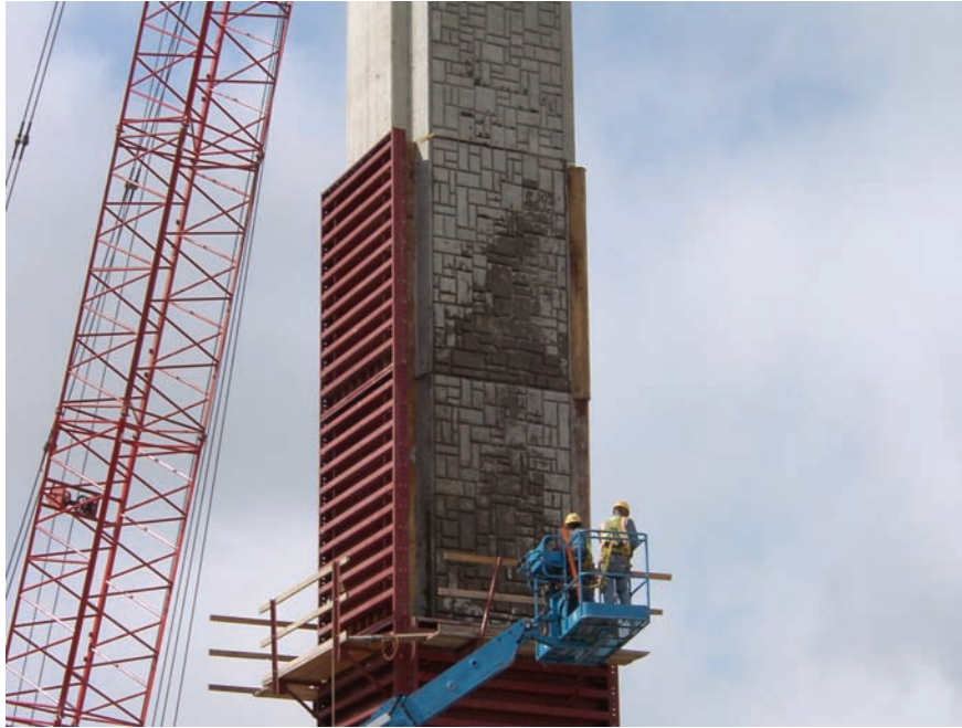
Figure 3.5 Rectangular Column during Form Removal and the Beginning of the Second construction stage (Riding 2007)
