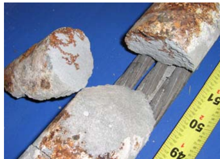
North Duct Grout
