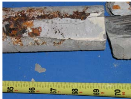
North Duct Grout
