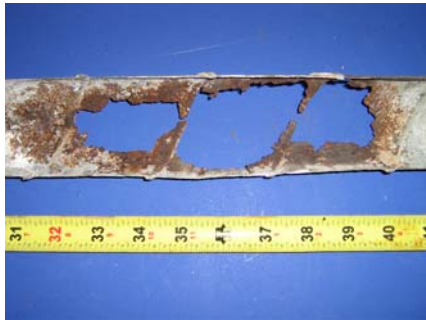
Top of North Duct
