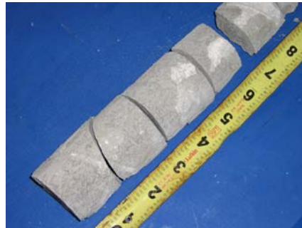
North Duct Grout
