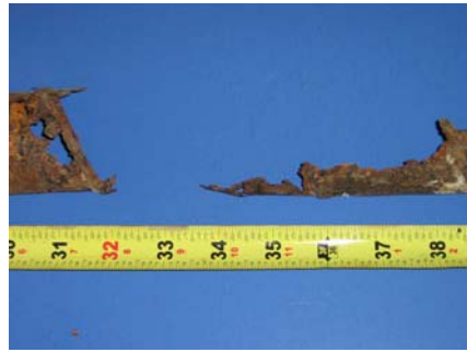
Top of North Duct
