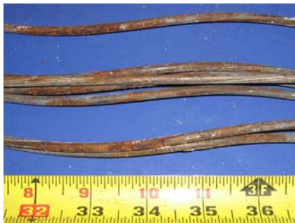
North Duct Strand
