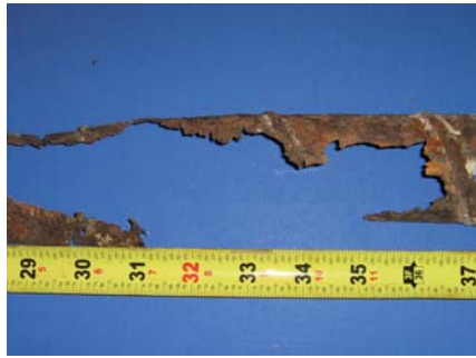
Top of South Duct
