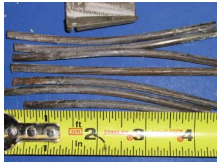
North Duct Strand
