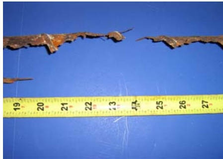
Top of South Duct
