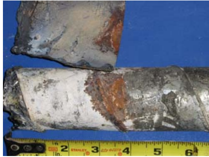
Top of South Duct
