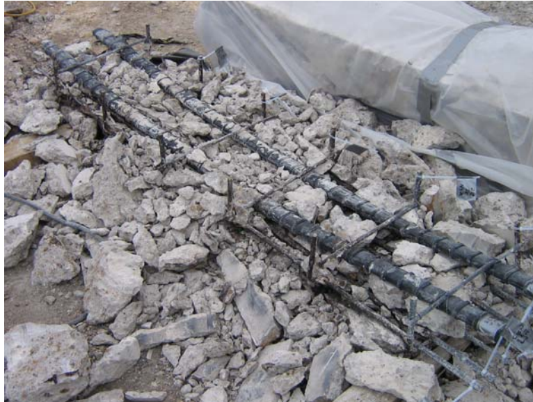
Figure 5.3: Post-Tensioning Ducts Before Removal from Center Block (Phase II Beam 2.12 Pictured)
