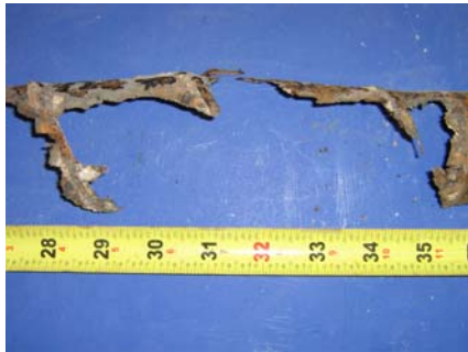
Top of South Duct
