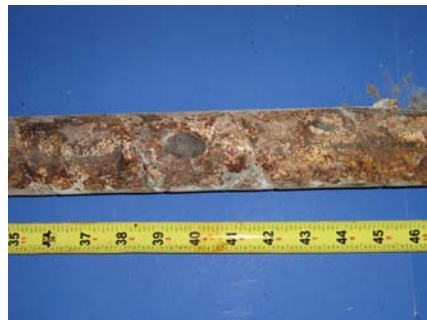
North Duct Grout
