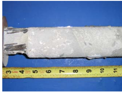
North Duct Grout
