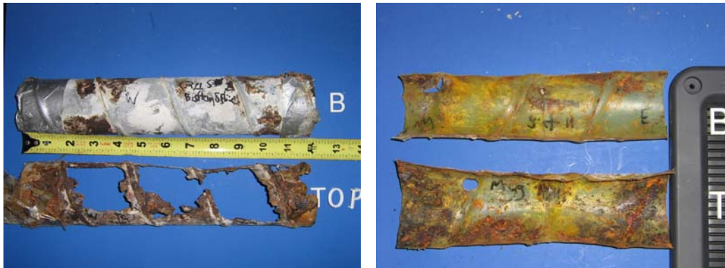
Figure 5.21: Beam 2.4 Duct Splices-South Duct Industry Standard Splice (Left) and North Duct Heat Shrink Splice (Right)
