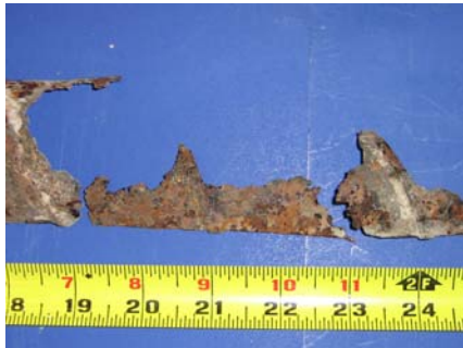
Top of South Duct
