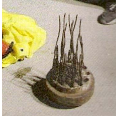
Figure 1.2: Corroded Anchorage (Bearing Plate with Strand Tails) 4
