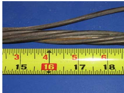
North Duct Strand
