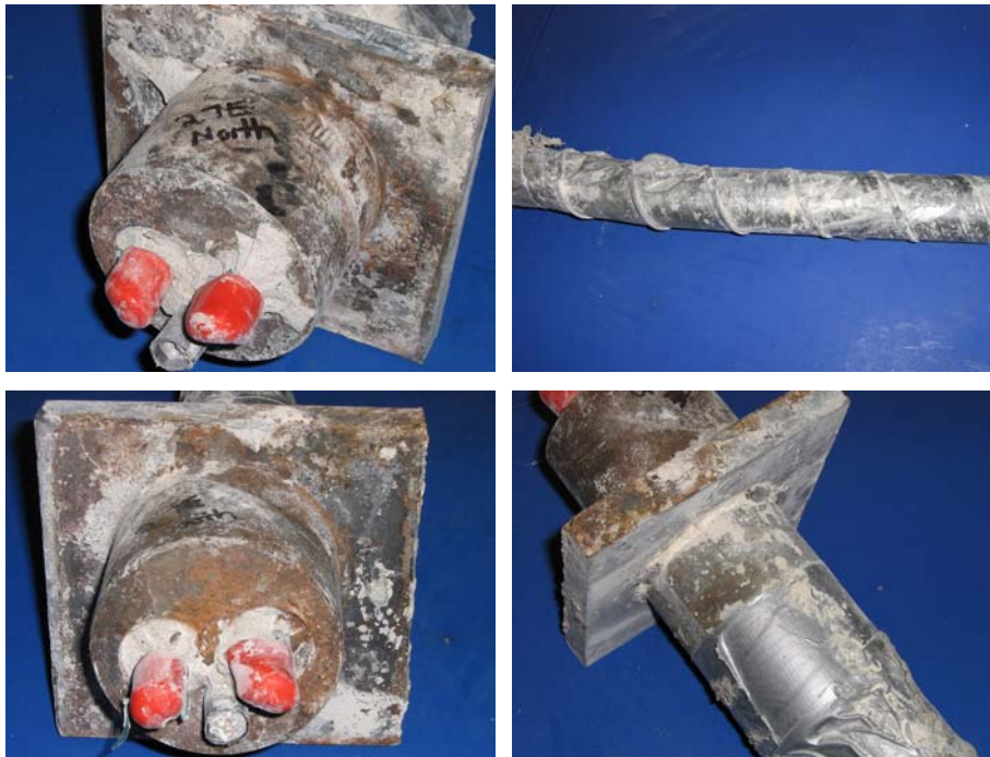
Figure 5.39: Beam 2.7 East End Anchorages (Dripped End): North Duct Anchorage (Top, Left and Right), and South Duct Anchorage (Bottom, Left and Right)
