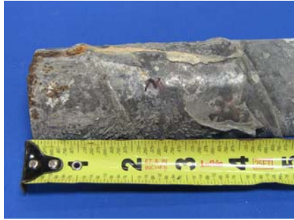
Top of South Duct
