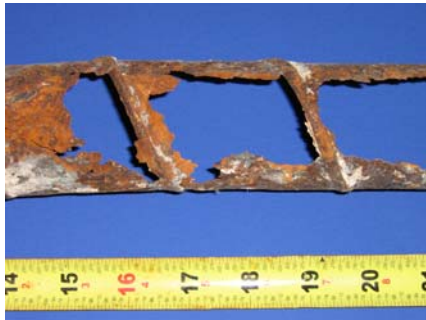
Top of South Duct
