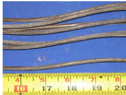
North Duct Strand
