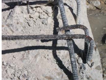
Figure 5.63: Beam 2.12-Corroded Stirrup in East End Anchorage Zone (Dripped End)
