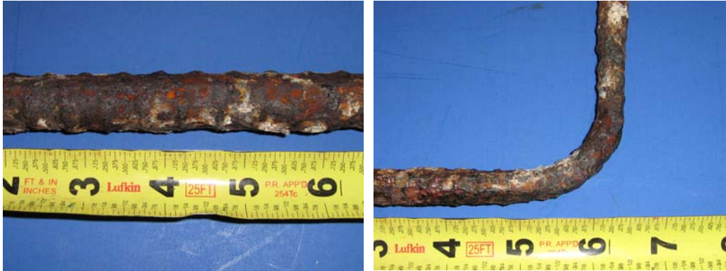
Figure 5.8: Beam 1.1 Autopsy Elements-Longitudinal Bar (Left) and Stirrup (Right)
