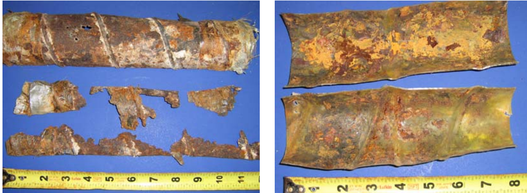
Figure 5.15: Beam 2.1 Duct Splices-South Duct Industry Standard Splice (Left) and North Duct Heat Shrink Splice (Right)
