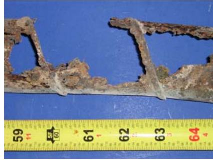
Top of North Duct
