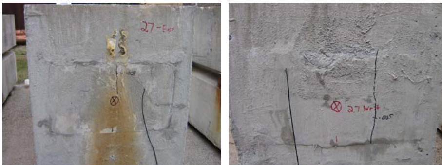
Figure 5.36: Beam 2.7 Anchorage Zones-East End (Left) with Dripper, and West End (Right) without Dripper
