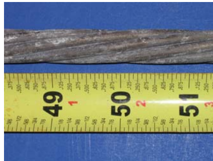
North Duct Strand
