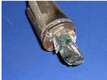
North Duct Strand With Wedges
