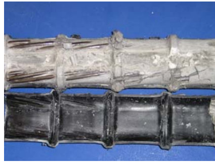
North Duct Grout (From Bottom)
