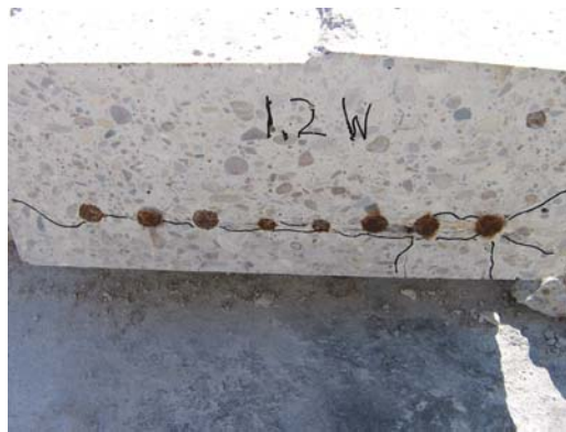
Figure 5.11: West End of Autopsy Block-Beam 1.2
