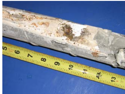
North Duct Grout
