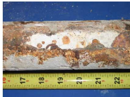
North Duct Grout
