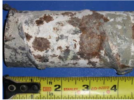
Top of North Duct
