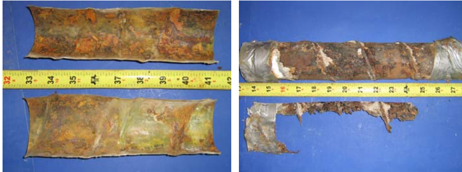
Figure 5.44: Beam 2.8 Duct Splices-South Duct Heat Shrink Splice (Left) and North Duct Industry Standard Splice (Right)
