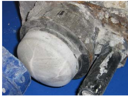
South Duct Grout Cap
