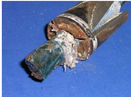
South Duct Strand With Wedges
