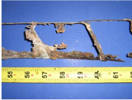
Top of South Duct
