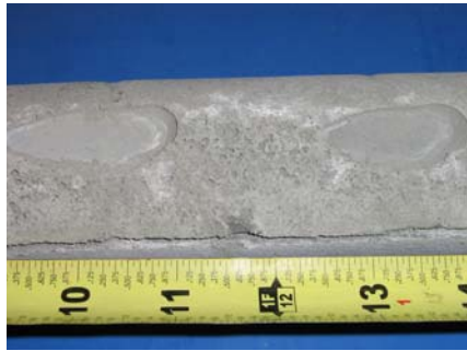
North Duct Grout
