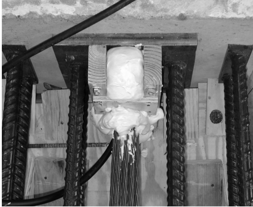
Figure 4-8 Sealing of Duct Ends
