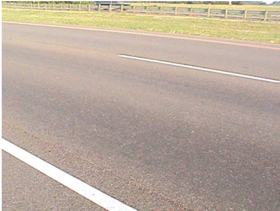
Figure B.1 Shallow rutting (<0.5 in) and flushing of asphalt on section 13010-1
