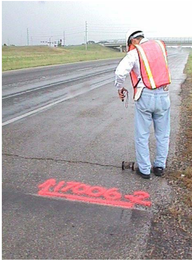
Figure 5.10 Beginning of section 17006-2 with a transverse crack on southbound SH 6
