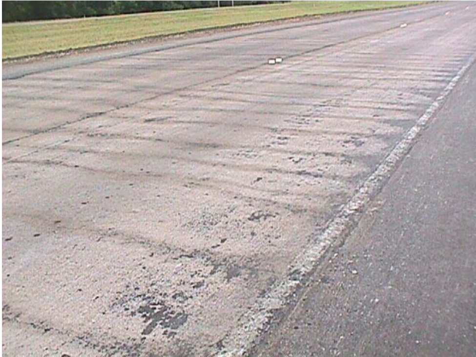
Figure B.2 Image of CRCP underneath the AC layer that was milled-off
