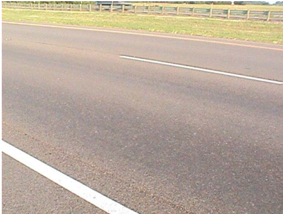
Figure 5.1 Shallow rutting (<0.5 in.) and flushing of asphalt on section 13010-1
