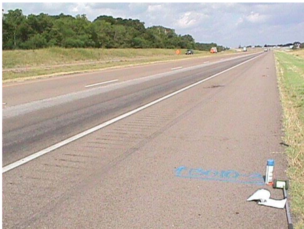
Figure 5.3 Image of rutted and flushed wheel paths of the outside lane
