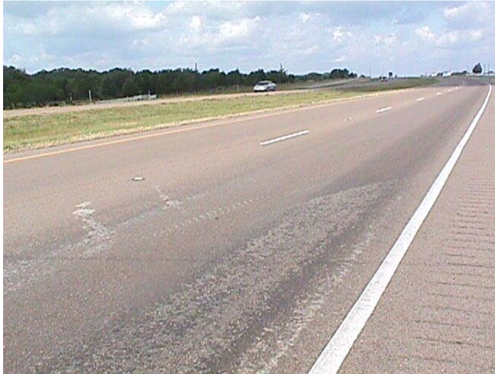
Figure 5.4 End of distressed asphalt layer area, section 13010-4
