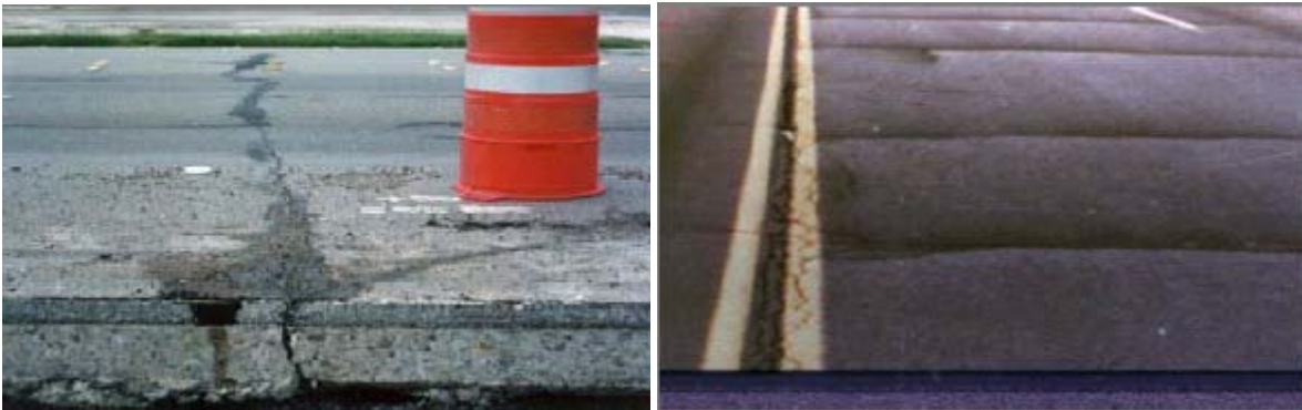
Figure 3.3 Reflection cracking
