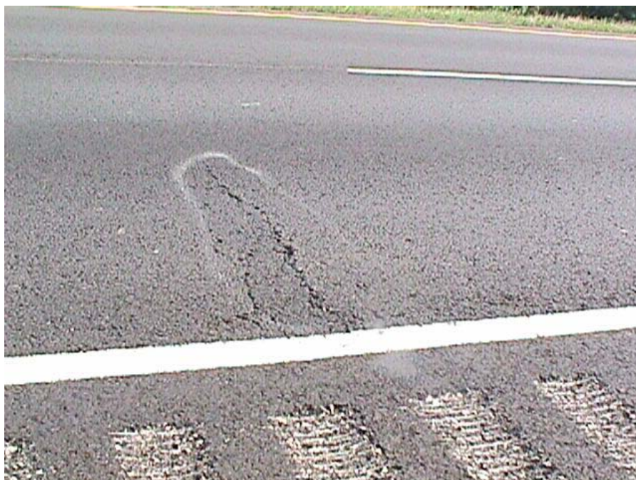
Figure 5.17 AC overlay delamination in section 19020-8
