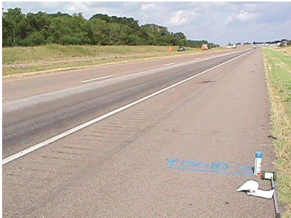
Figure B.3 Image of rutted and flushed wheel paths of the outside lane
