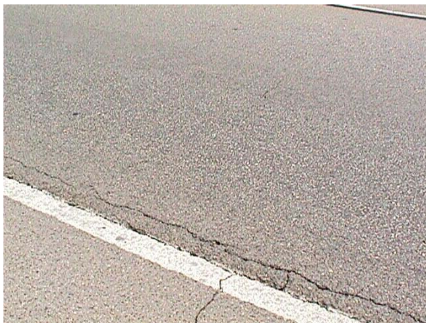
Figure 5.9 Longitudinal crack next to the shoulder in section 17006-1 on SH 6 in Brazos County
