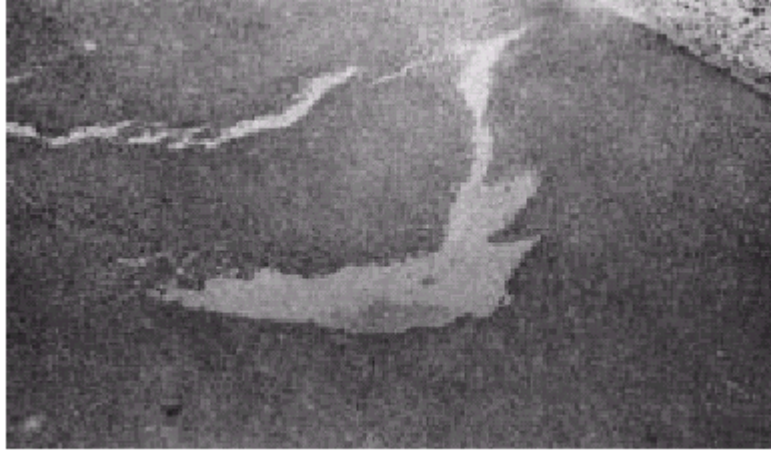
Figure 3.4 Slippage cracking
