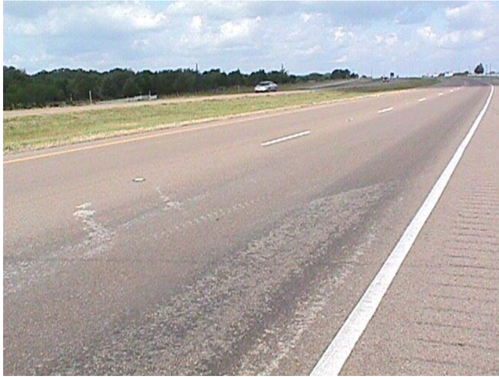
Figure B.4 End of a distressed asphalt layer area, section 13010-4
