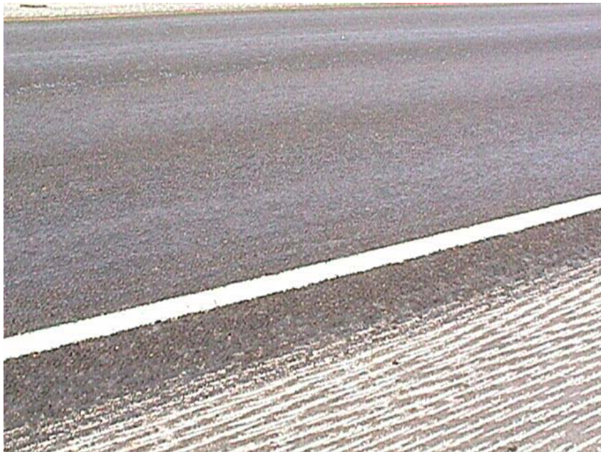
Figure 5.7 Section 17045-3, still showing non-resurfaced shoulder
