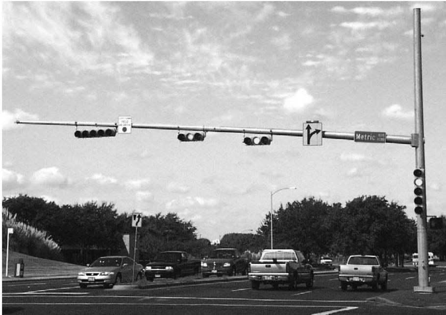
**Figure 1.1 Typical Cantilever Mast-Arm Traffic Signal Support Structure**
