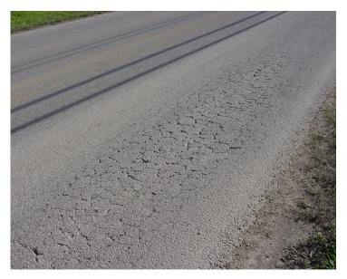
Figure 1. Fatigue Cracking
