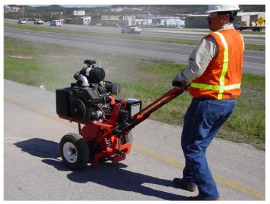
Figure 8. Crack Routing Procedure
