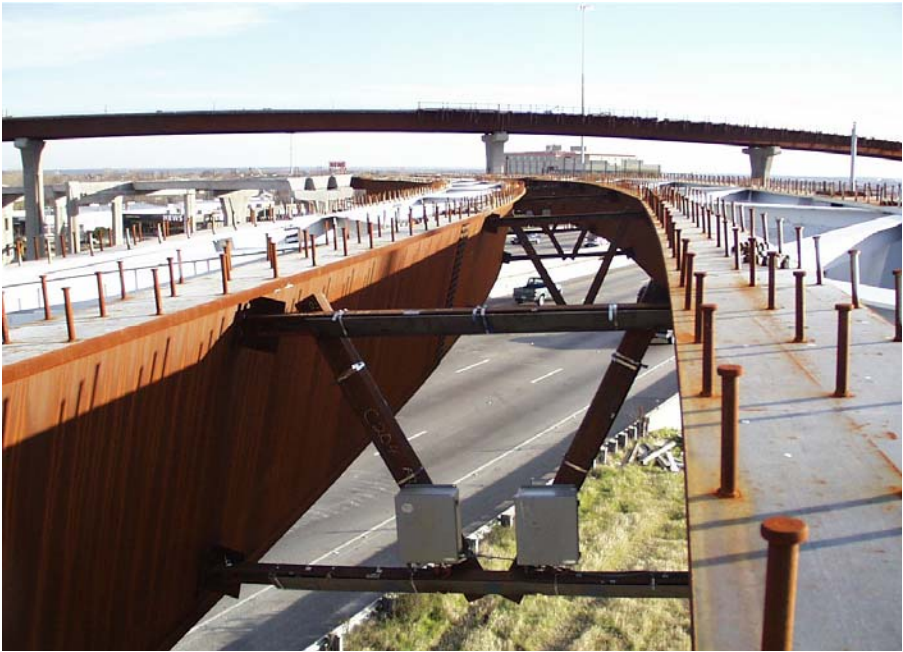
Figure 6.3 External Diaphragm #11 -- Looking South (Cheplak, 2001)
