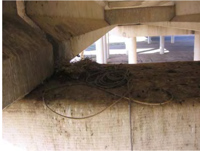
Figure 4.8 Location of embedded probe in Structure 8
