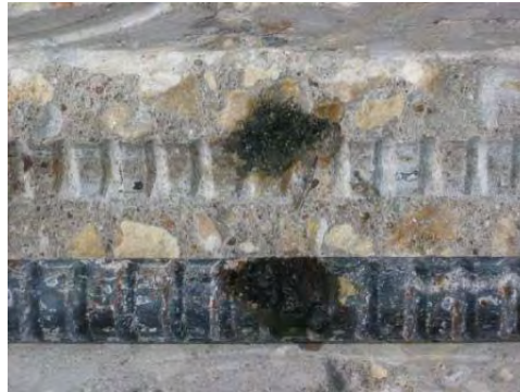
Heavy localized rusting on rebar A.
