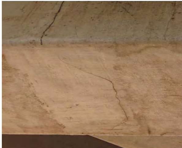
Figure 4.6 Crack on underside of bent on Structure 5
