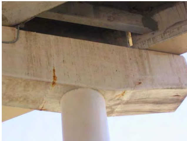
Figure 4.4 Rust staining on bent, Structure 1
