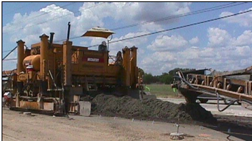
Figure 1-3: A typical concrete placement process where a slipform paver is used
