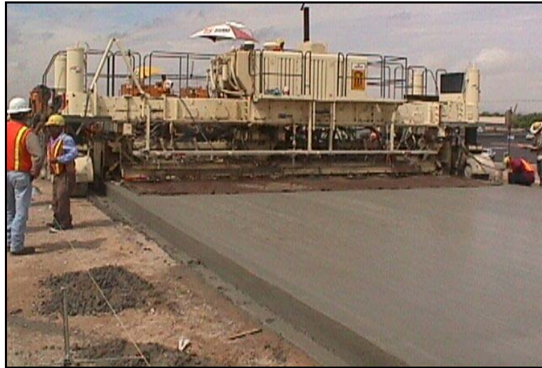
Figure 4-21: Photograph of construction operations on Loop 375 in El Paso, August 2000
