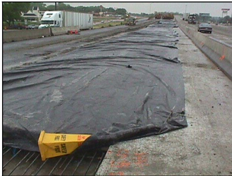
Figure 4-6: Newly paved pavement protected against rainfall, Dallas, May 2000
