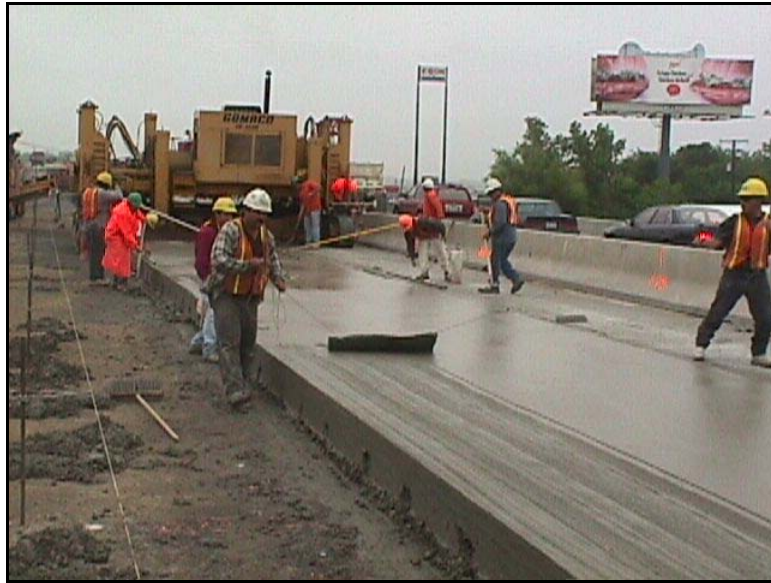
Figure 4-5: Photograph of construction operations on IH 45 in Dallas, May 2000
