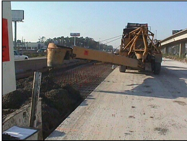
Figure 4-28: Photograph of construction operations on US 59, Houston, October 2000
