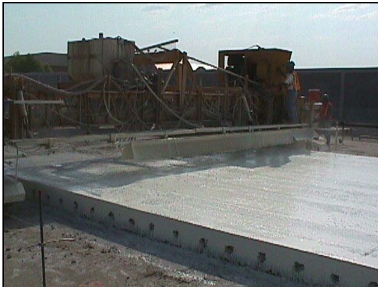
Figure 4-11: Photograph of construction operations used on SH 190 in Dallas, August 2000
