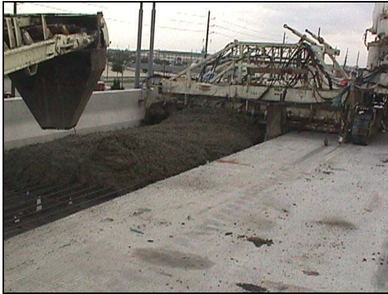
Figure 4-8: Photograph of construction operations used on IH 45 in Dallas, May 2000
