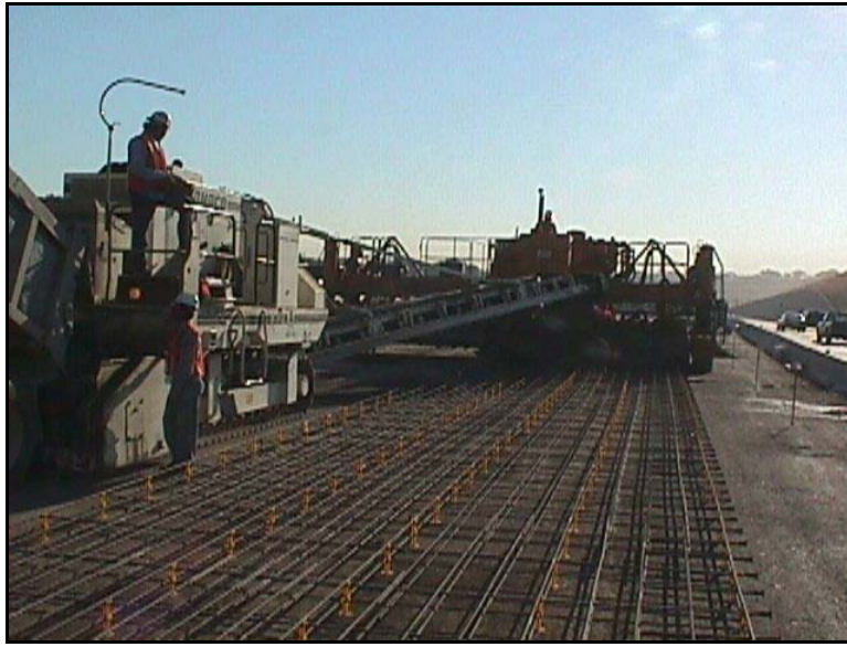
Figure 4-24: Photograph of construction operations on IH 30, Dallas, September 2000
