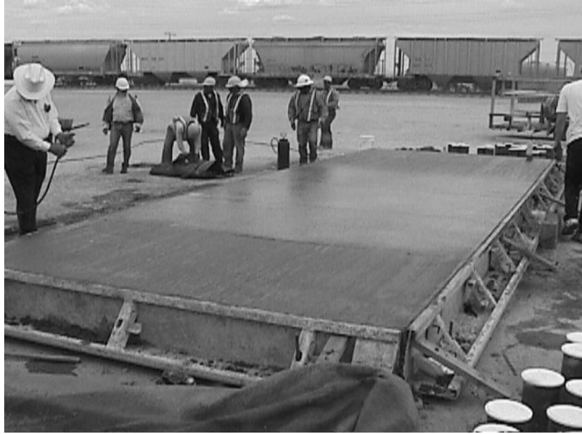
Photo 4.4 Slab after Concrete Placement, Burlap Finish, and MMF Application
