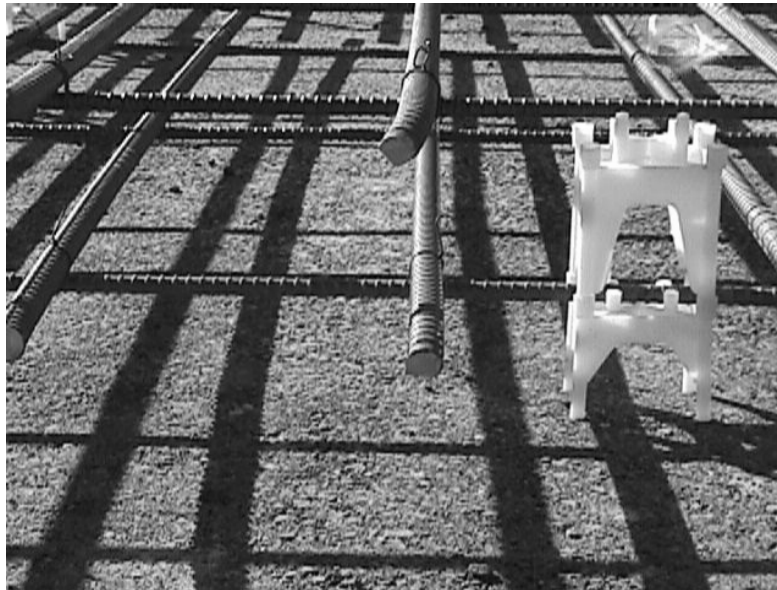
Photo 4.2 Closeup of Double Mat Reinforcement Setup Prior to Concrete Placement
