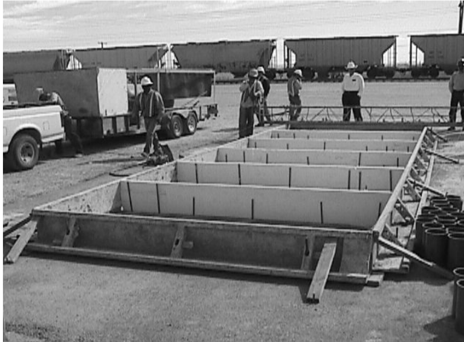
Photo 4.3 Formwork and Foam Separation Prior to Concrete Placement
