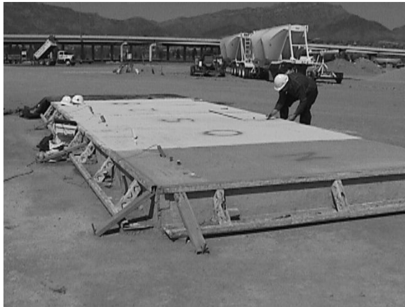
Photo 4.5 Slab after Concrete Application of Curing Compound and Plastic Sheeting
