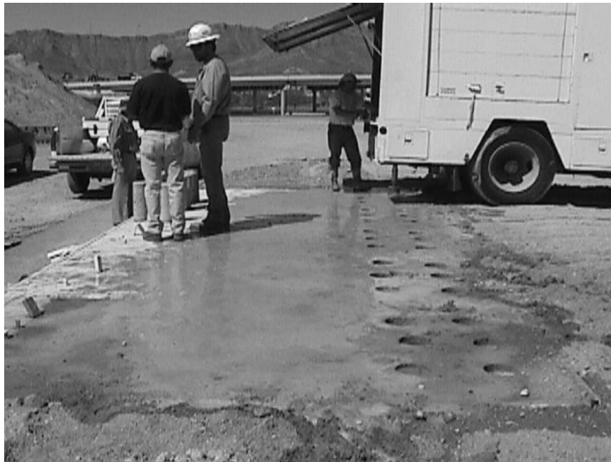
Photo 4.6 Slab after 3-Day Coring and Construction of Ramp for Coring Truck
