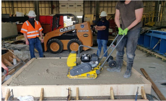
Compaction of cement stabilized bases
