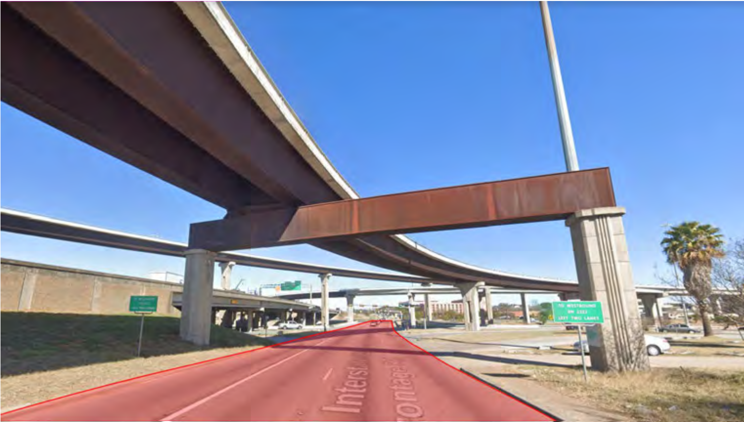
Box straddle cap supporting twin tub girders on I35N & US290 (Google Maps)
