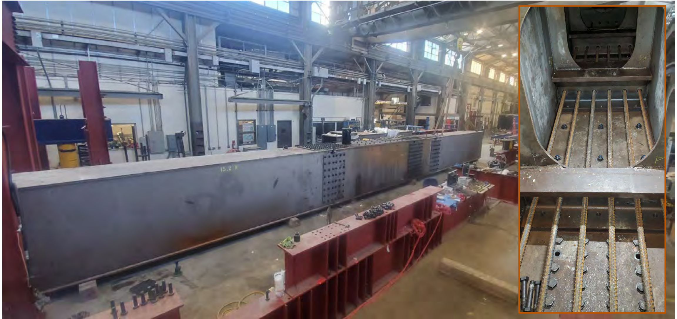
Assembly of Specimen A to be tested with addition of high-strength bars
