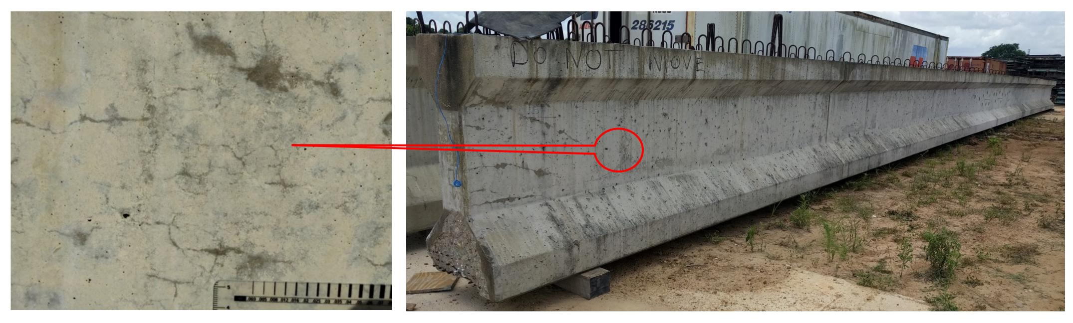
Fig: Typical pre-stressed girder showing surface microcracking
