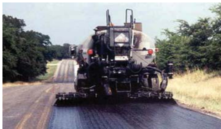
Pavement Maintenance in Action: Application of Fog Seal
