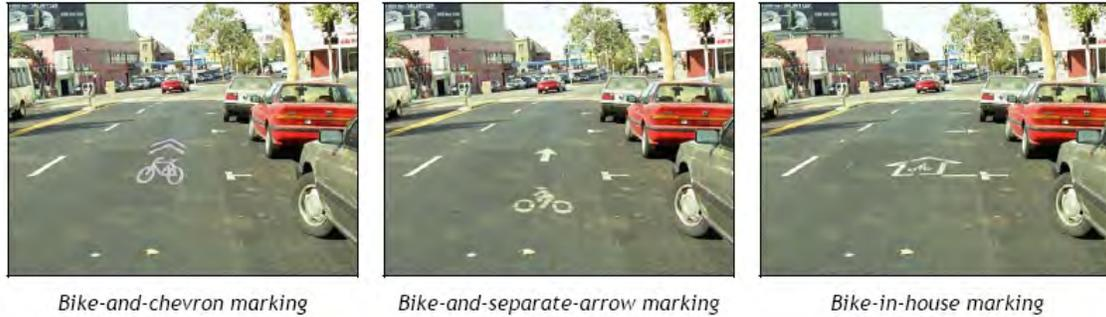
Figure 2.8: Photographs of Pavement Markings Used in Stated Preference Survey
