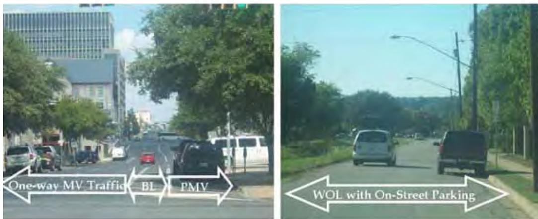
*Figure 3.4: Examples of one-way streets with BL (left) and WOL (right) and motor vehicle parking on-street*
