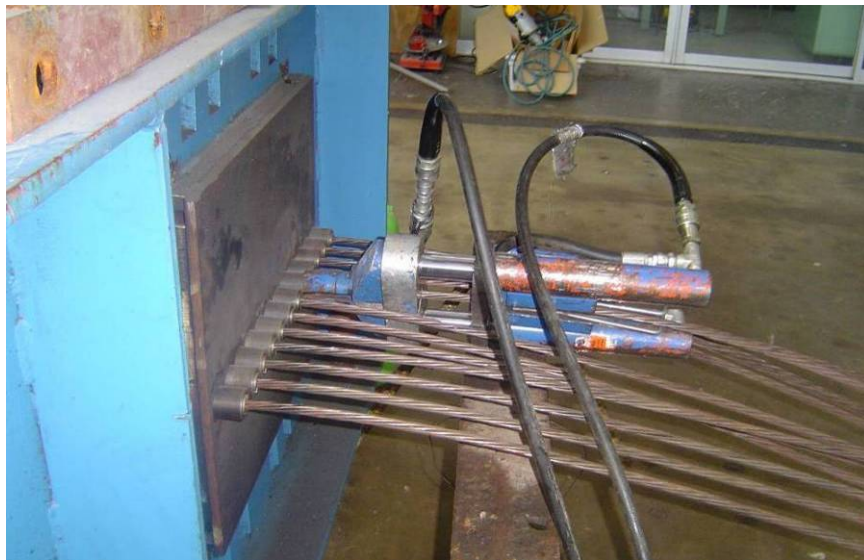
Figure 3-26 Single strand stressing operation.
