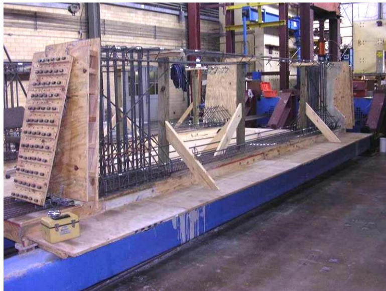
Figure 3-14 AASHTO Type IV beam during fabrication.
