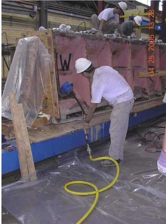
Figure 3-28 Form vibrators used to consolidate concrete.
