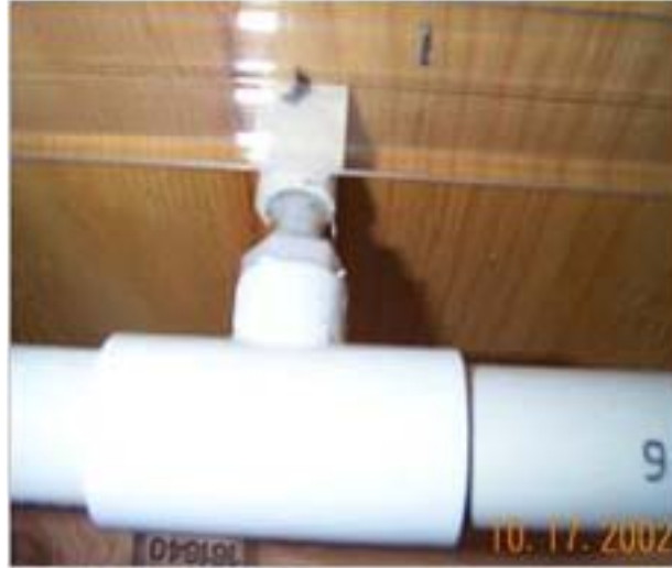
Figure 9. Underdrain inlet.
