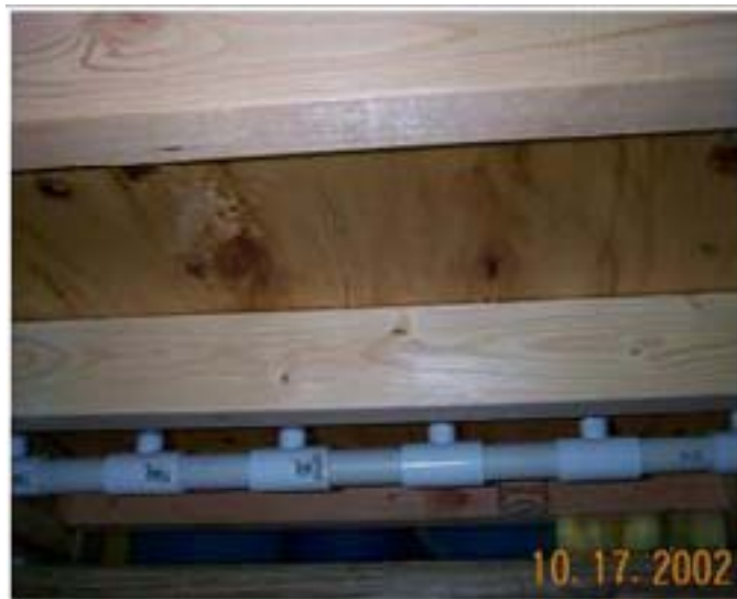
Figure 10. Underdrain collection manifold.
